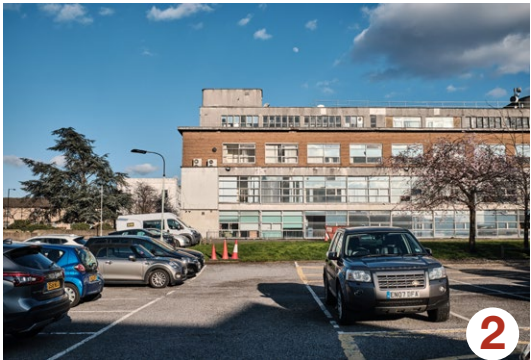
Car Park Site
