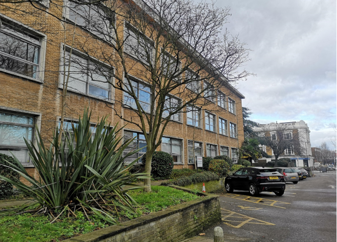
Image of existing frontage
