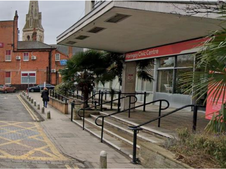
Figure 9 – Replacement Handrails
