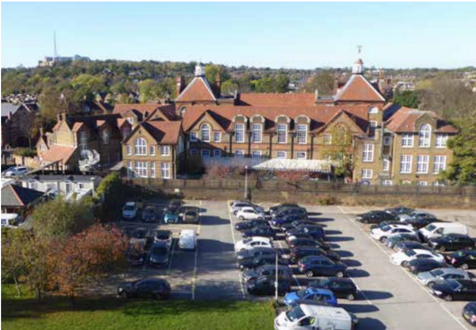
Figure 4.8 View of rear elevation of Trinity School from the Site (2018)
