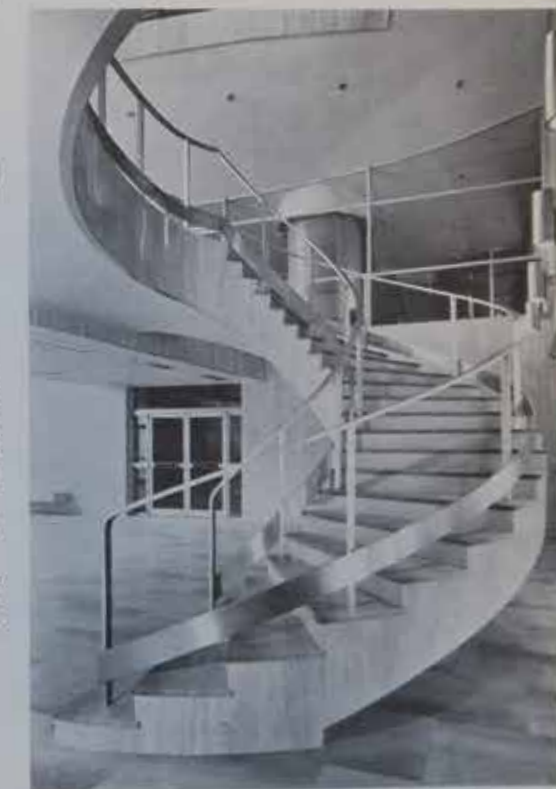
Above: circular staircase in the entrance hall with serpegiente marble and anodised aluminium balustrading
