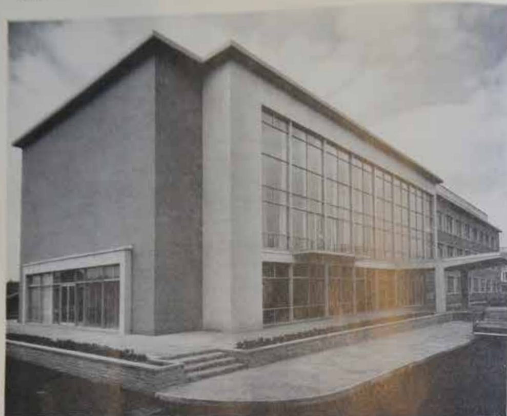
East elevation with the canopy over the entrance and the full height windows to the council chamber
