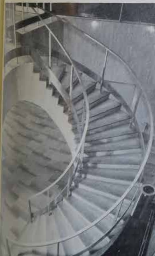
A view across the bridge that spans the entrance to the council chamber. below: The spiral staircase from the hall to the bridge. right: Opal perspex sheets in office corridor
