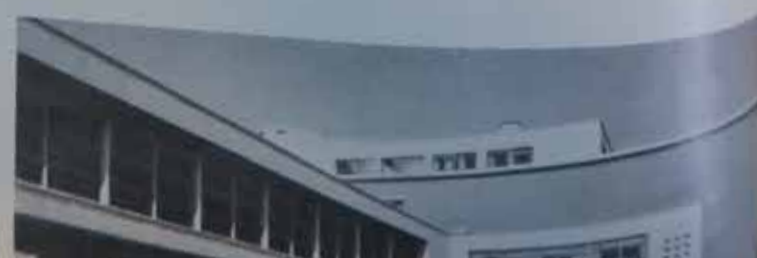
View from south-west
