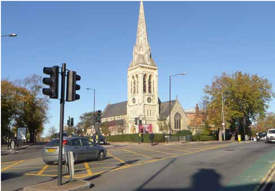
Figure 4.9 View of Church of St. Michael from junction of High Road and Bounds Green Road (2018)
