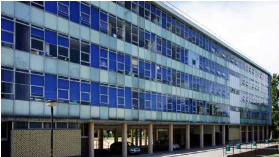
Figure 5.1 Elliott School in Putney, LB Wandsworth (now Ark Putney Academy) prior to refurbishment
