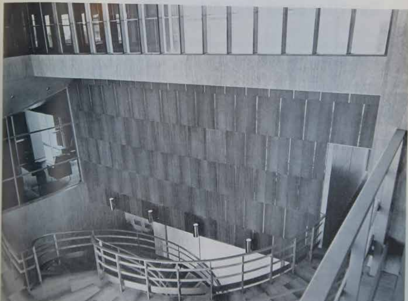
The helical main staircase, which rises to the bridge giving access to the Council Chamber, has a mean radius of 5 ft. 3 in. and is 5 ft. in width. In rising it traverses 270^{\circ} and continues with a radius of 14 ft. 6 in. until it reaches the first floor, having in plan a shape rather like a figure six. The wall above the staircase has panels of elm-veneered plywood, divided by vertical strips of polished brass (a detail is given above, right)
