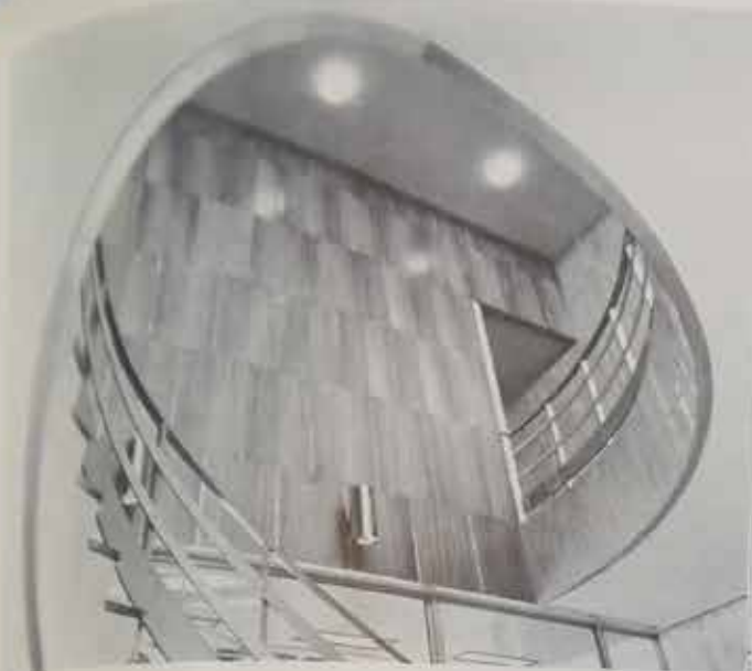
The helical main staircase, which rises to the bridge giving access to the Council Chamber, has a mean radius of 5 ft. 3 in. and is 5 ft. in width. In rising it traverses 270^{\circ} and continues with a radius of 14 ft. 6 in. until it reaches the first floor, having in plan a shape rather like a figure six. The wall above the staircase has panels of elm-veneered plywood, divided by vertical strips of polished brass (a detail is given above, right)
