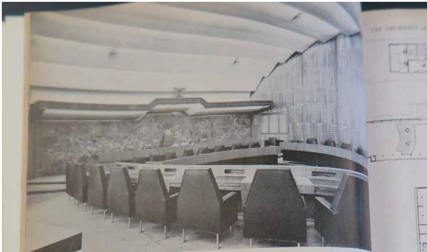
Top, interior of the council chamber. The wall behind the Mayor's dais is faced in Vert de Fray marble. Side walls are veneered in elm with brass edge strips. Below, view from the public gallery
