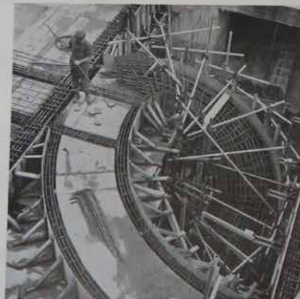
The reinforcement to the circular stair
