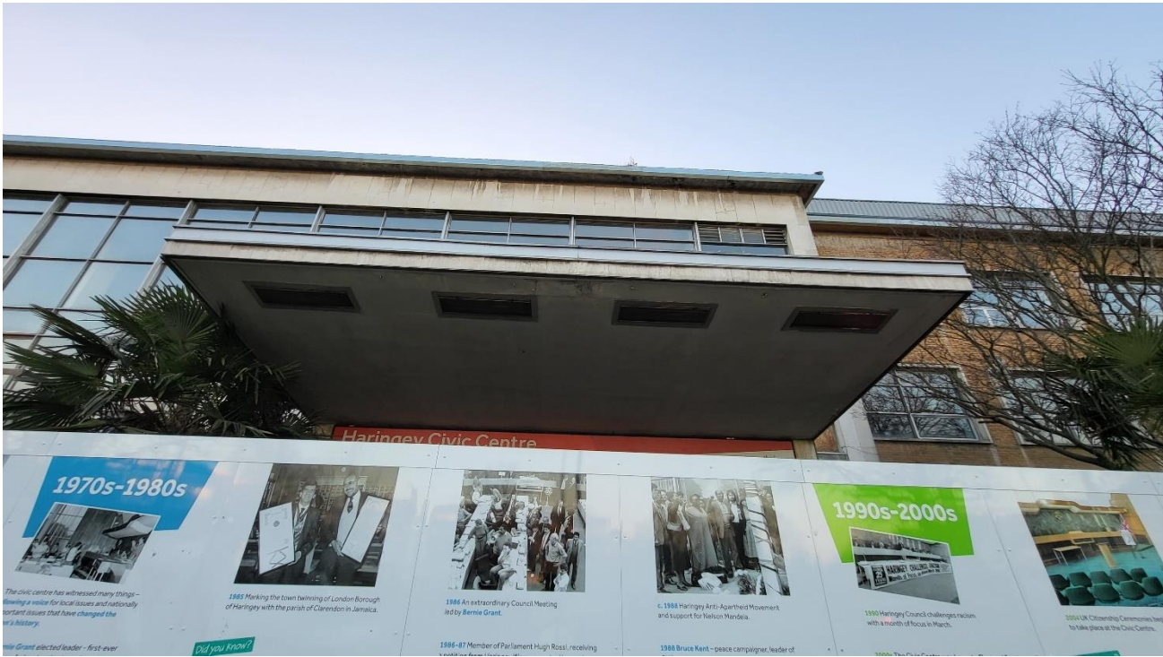
Figure 2.4 – View 4 West – Haringey Civic Centre, entrance canopy.
