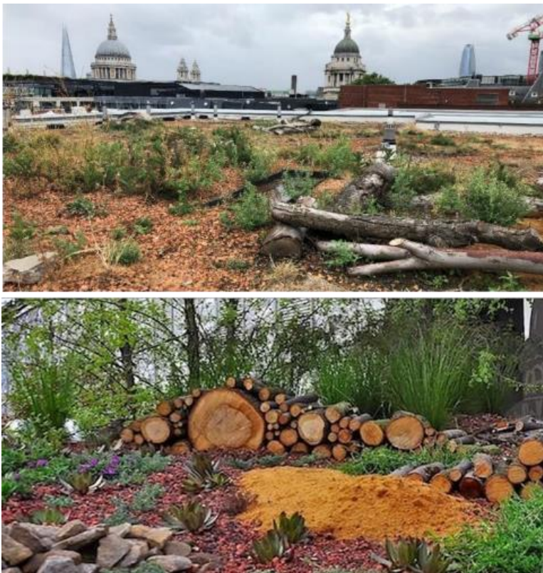
Figure 5.2 Log piles on a biodiverse living roof
