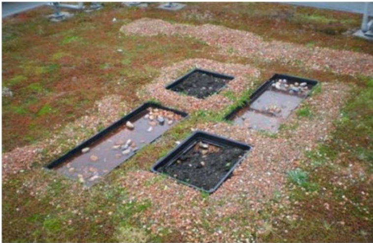
Figure 5.5 Water and mud trays embedded within the substrate of a green roof. Photo credit: Edward Mayer, Swift Conservation Trust
