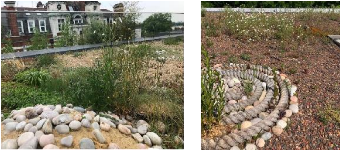
Figure 5.3 Rope coils on biodiverse living roof
