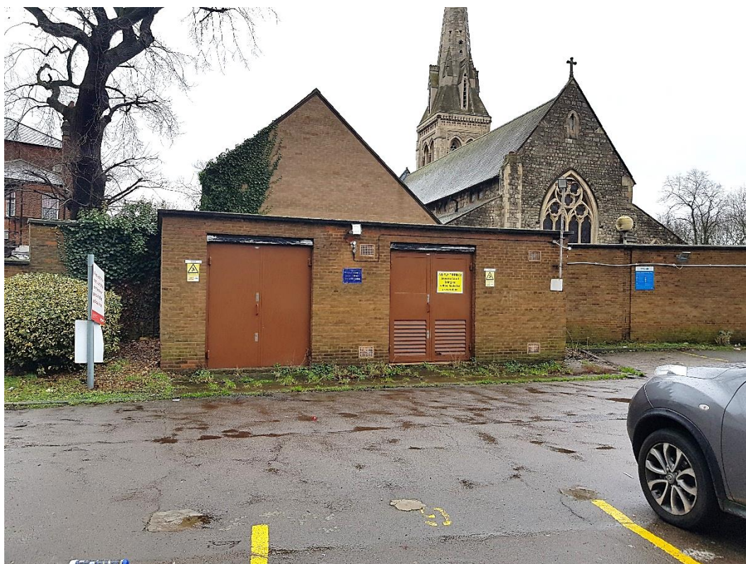
Figure B.2 Building 2, west side
