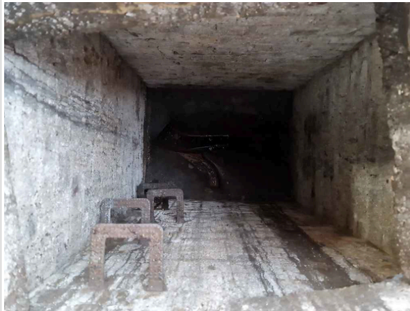
MH3/SW TOP VIEW
