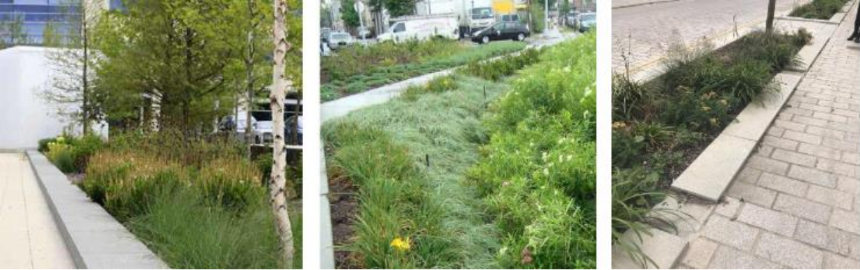
Figure 5-3 Examples of bioretention systems/raingardens.
