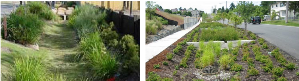
Figure 5-2 Examples of swales in residential developments.
