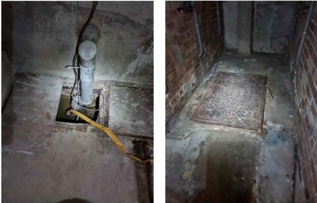
Figure 7-3 Existing manholes in the Civic Centre basement. Left: Manhole 1 (ref MH7/FL in CCTV survey) and Right: Manhole 2 (ref MH6/FL in CCTV survey).
