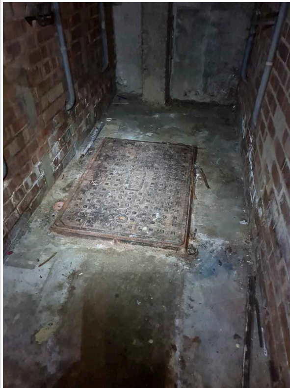
MH6/FL IN THE BASEMENT AREA
