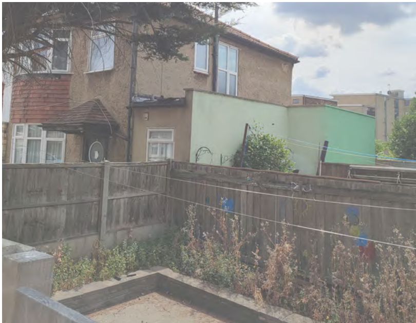
Existing side extension
