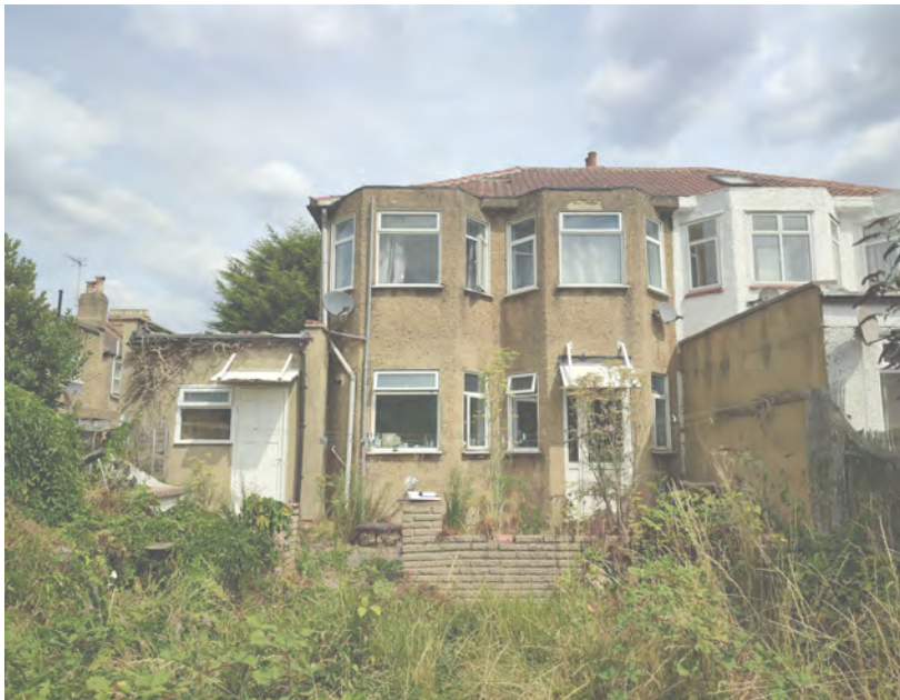
Rear elevation from garden area, showing neighbouring rear extension to right
