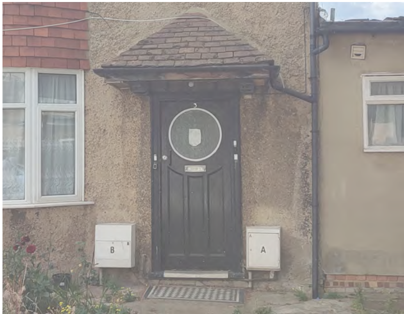
Front communal entrance door
