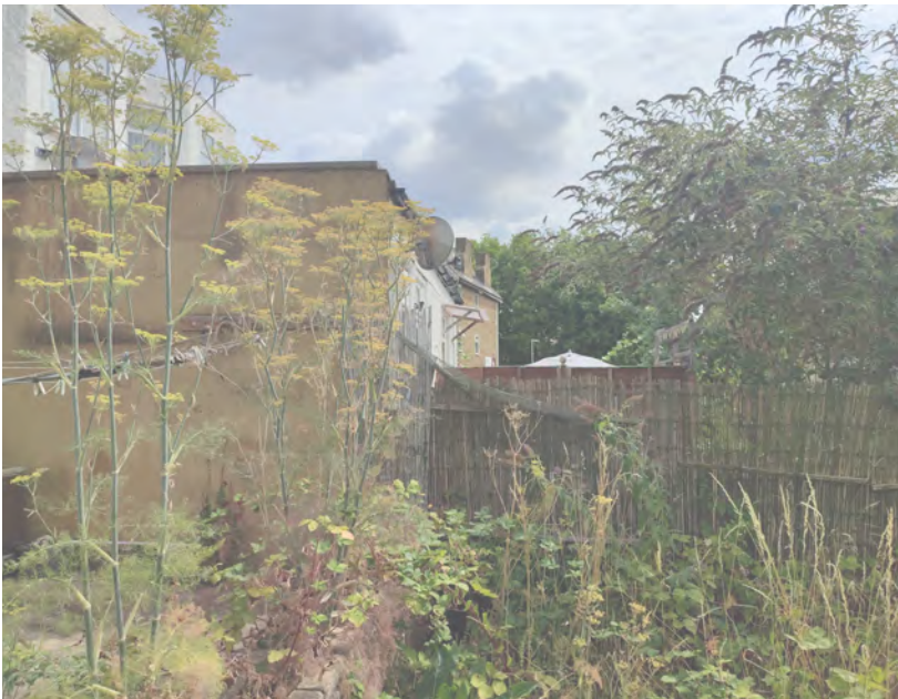
Large neighbouring rear extension, image from garden
