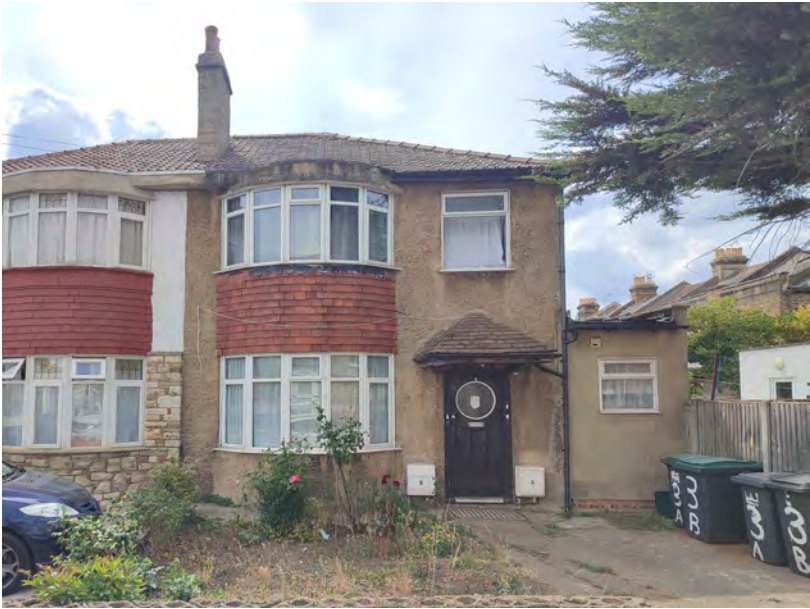
Front Elevation Photograph showing material pallet
