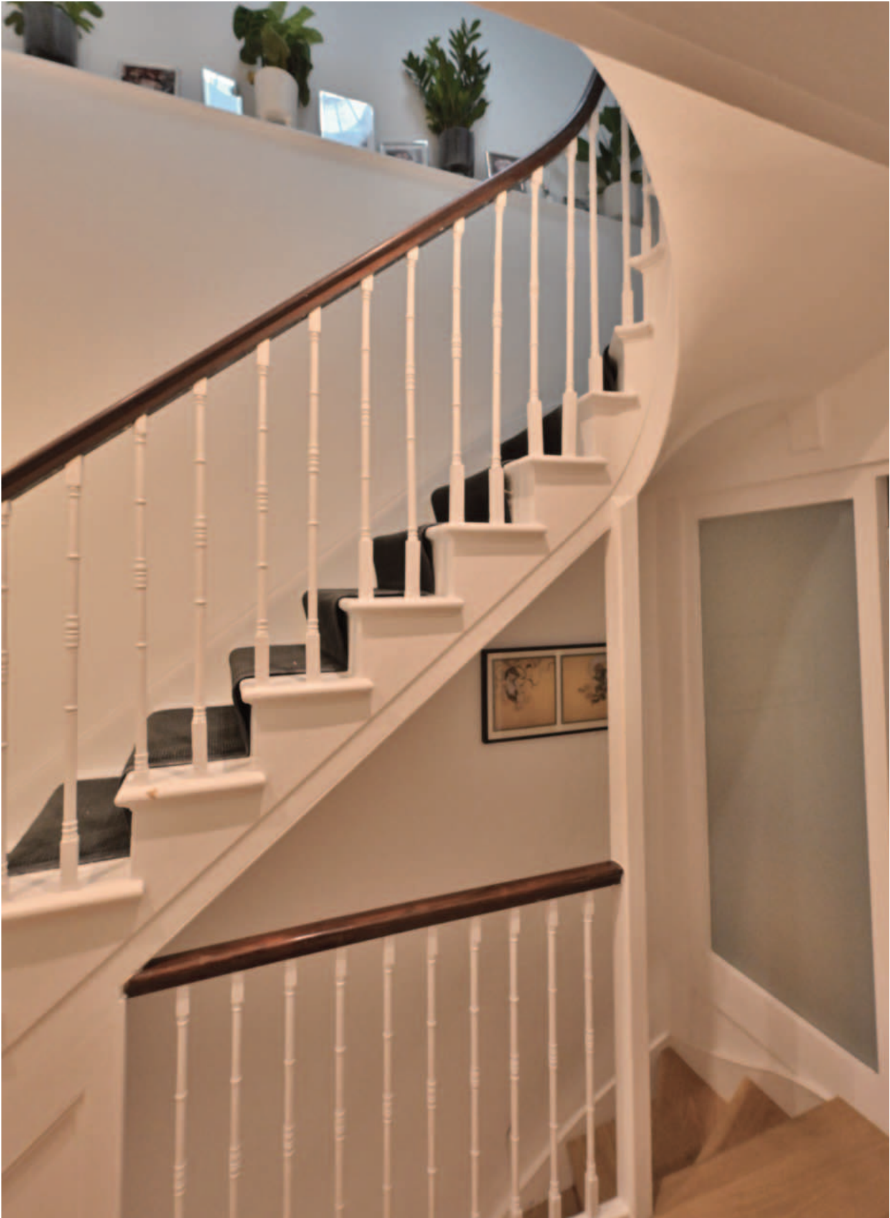
Fig. 27. The basement stair has been opened up and a section of balustrade a glazed panel and a crude rectangular newel post replaces the boarded enclosure that would have separated off the basement rooms.
