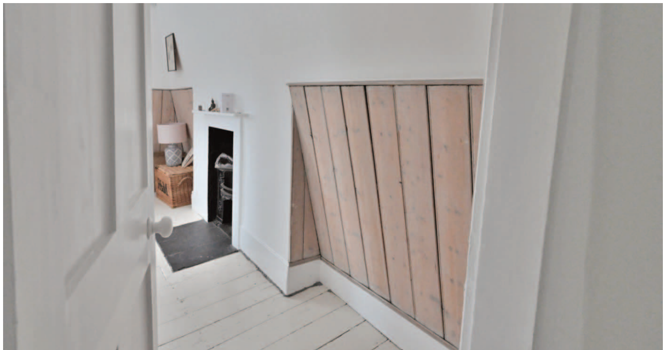
Fig. 43. Detail of the timber boarding below dado level within the south room. The fireplace retains its original hob-grate, mantelsheaf and hearth.
