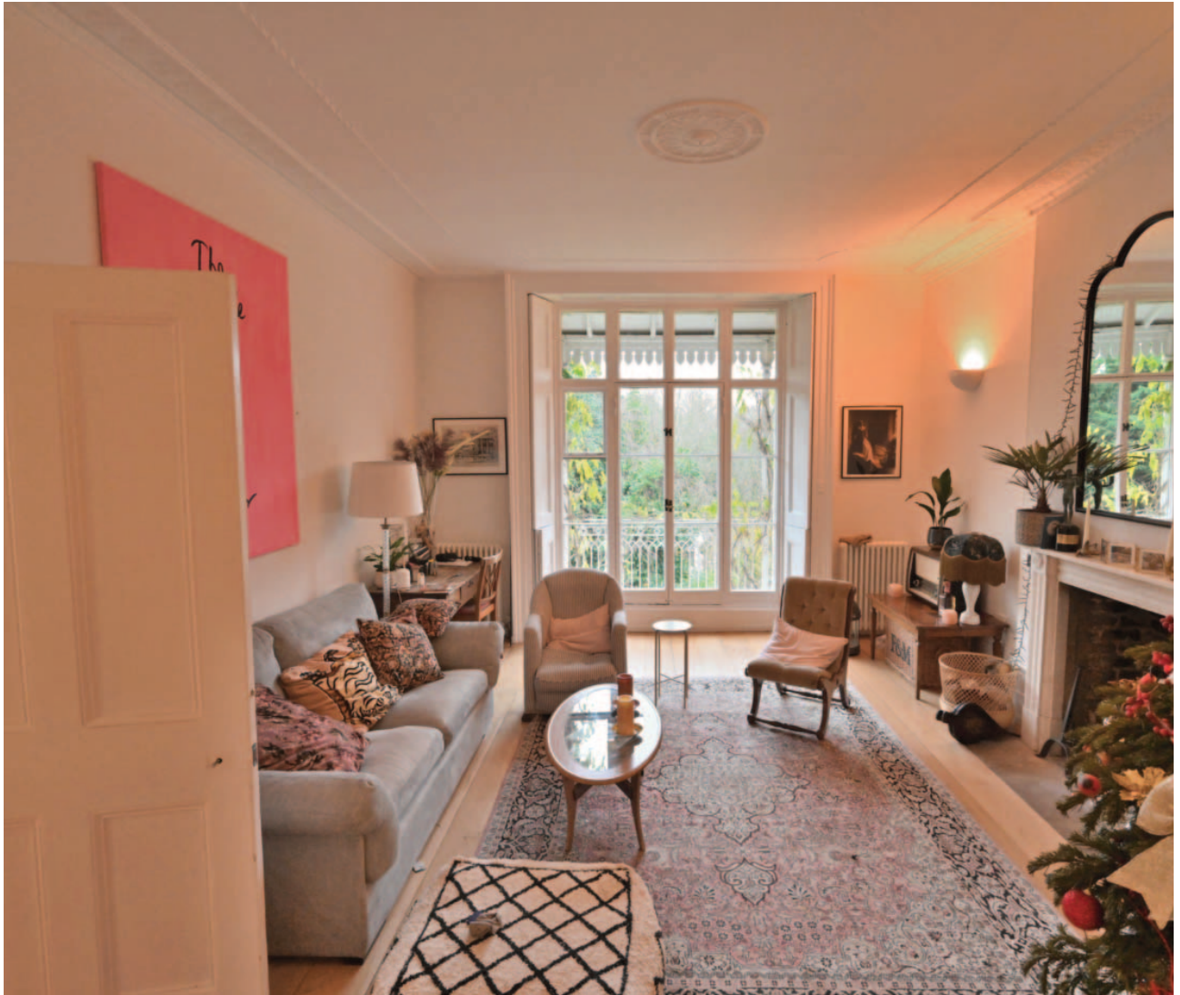
Figs. 23. The principal ground floor reception room with its restrained ceiling rose and foliate and beaded cornice. The inner band of elongated bellflowers on the ceiling bed is a later introduction. The marble fireplace and hearth appear to be original but reset on the modern overboarded floor.
