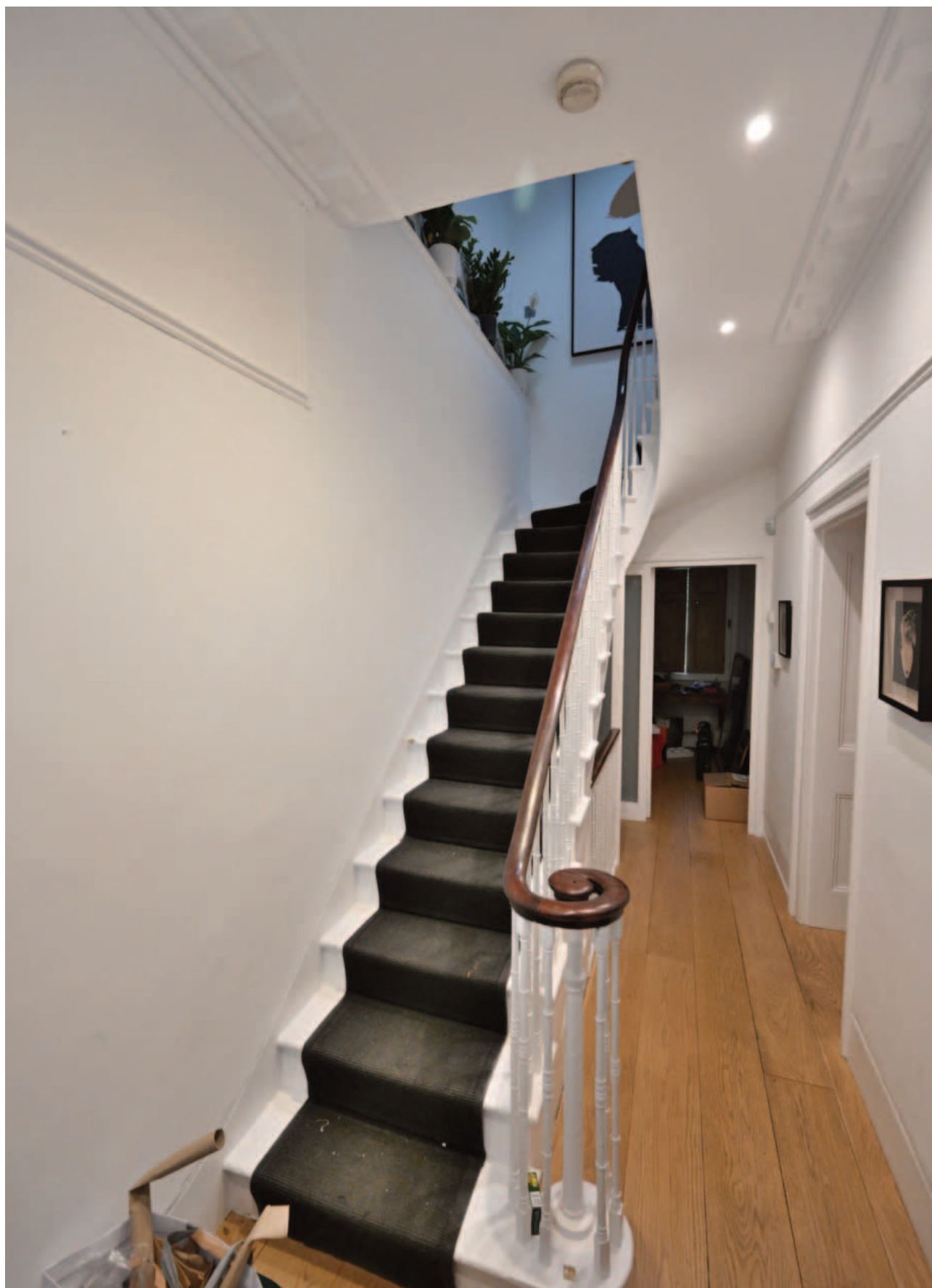
Fig. 20. The entrance hall with its dentilled cornice and elegant staircase. On the right is the door into the principal reception room with its fine architrave and panelled lining. The floor has modern overboarding.
