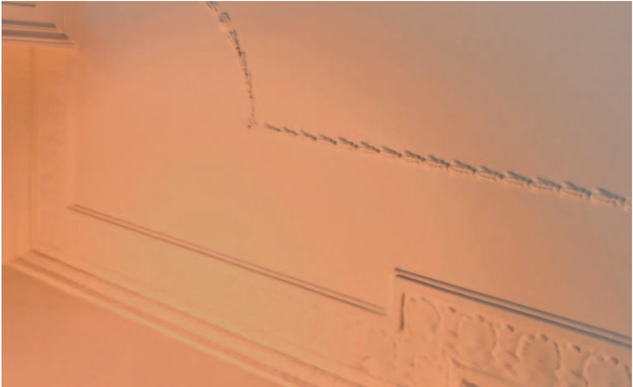
Fig. 24. Detail of the heavily overpainted ceiling cornice, with the later foliate addition on the ceiling bed.
