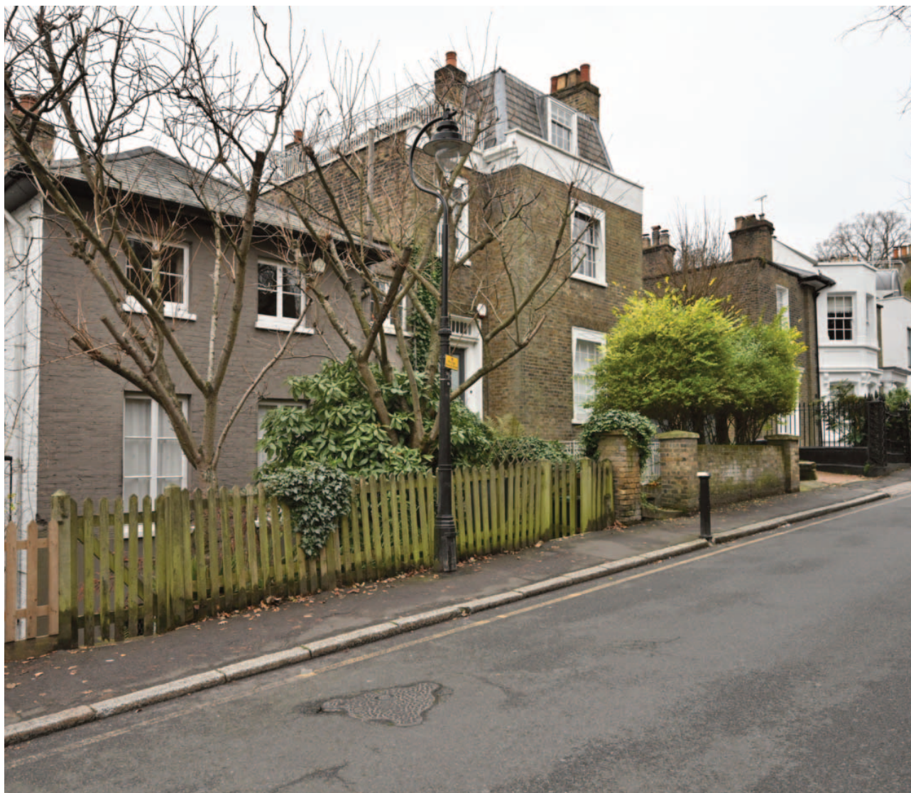
Fig 2. Nos 10 and 12 Wood Lane are separately listed at grade II (as is the simple brick boundary wall). The unlisted No 14 in the foreground (left) is mentioned as having group value with Nos 10 and 12.
