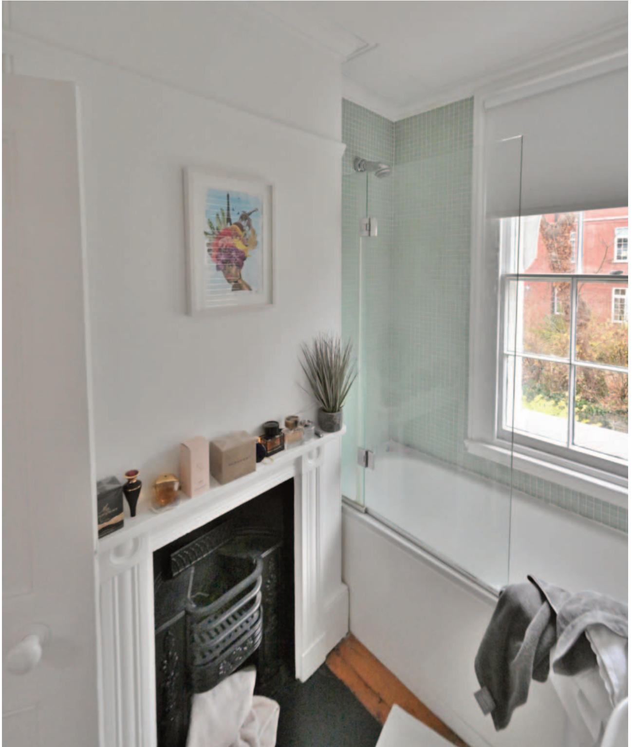
Fig. 37. The small front bathroom opening off the staircase has a small mid 19th century hob grate suggesting that it was originally a dressing room or small bedroom.
