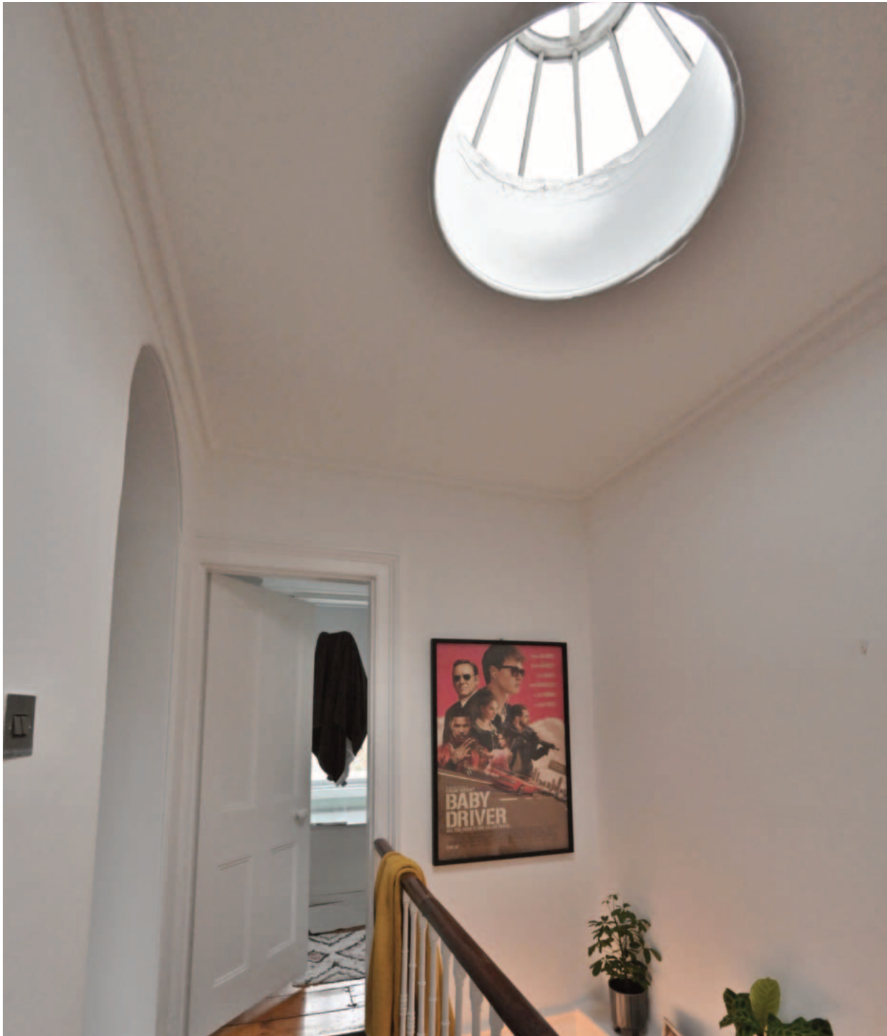
Fig. 34. The first floor landing with its simple cornice is lit by a historic skylight in the flat roof of the east wing. A small bathroom occupies the front room and the architrave and door match the detailing elsewhere.
