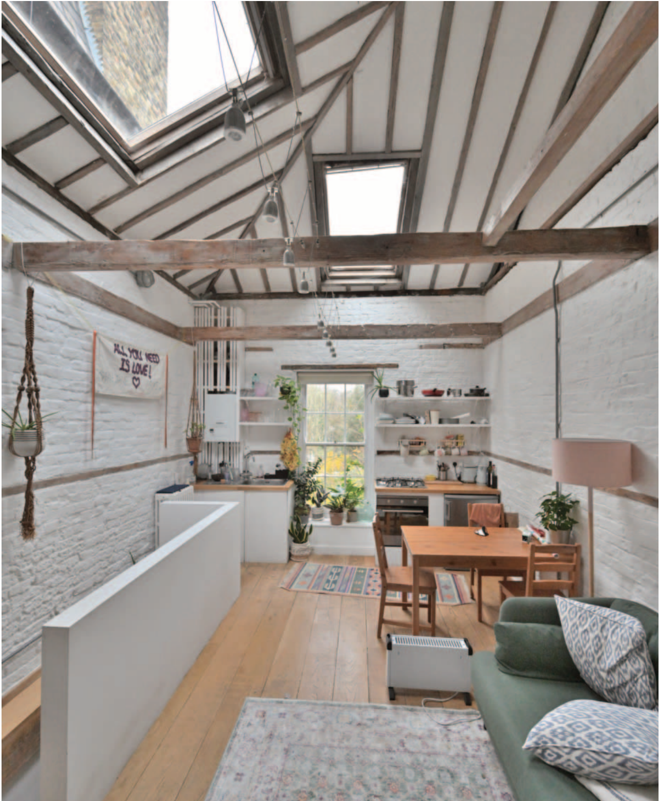
Fig. 44. The upper floor residential conversion within the outbuilding. A lath and plaster ceiling would have concealed the roof structure whilst the tall window in the rear wall may have held a hoist door.
