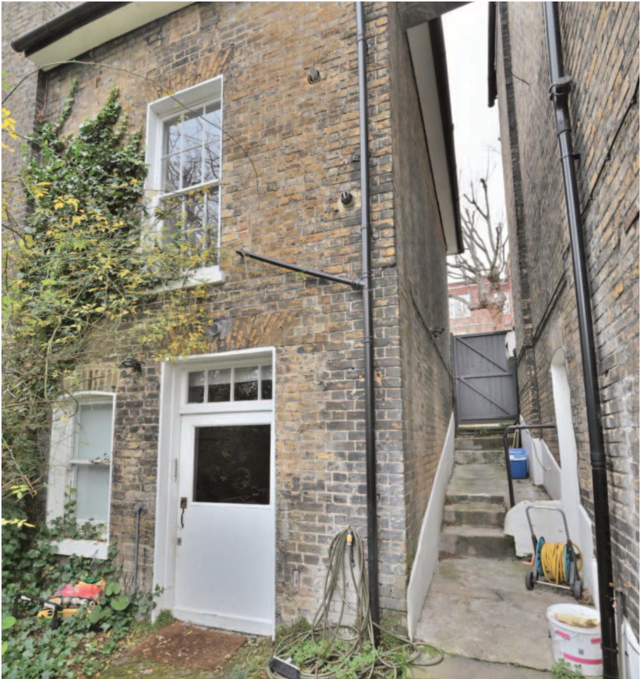
Fig. 14. The tall former stable door and later window (with the arched brick head) at ground floor level. The low wall adjacent to the side door of the main house was presumably to keep out rainwater from the path.
