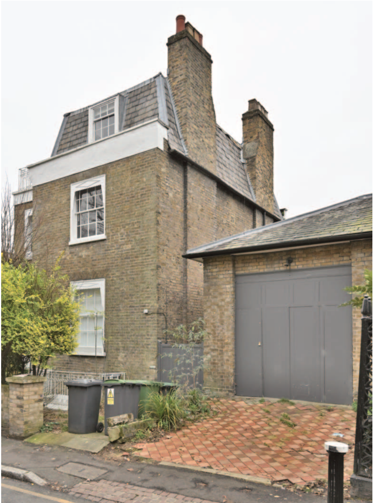
Fig 10. The west elevation of the main house with its two external stacks. Separated by a narrow path to the rear garden and tradesman's entrance is the two storey former coach house and workshop. The building reads as a single storey hipped roofed extension to the adjacent No 10.
