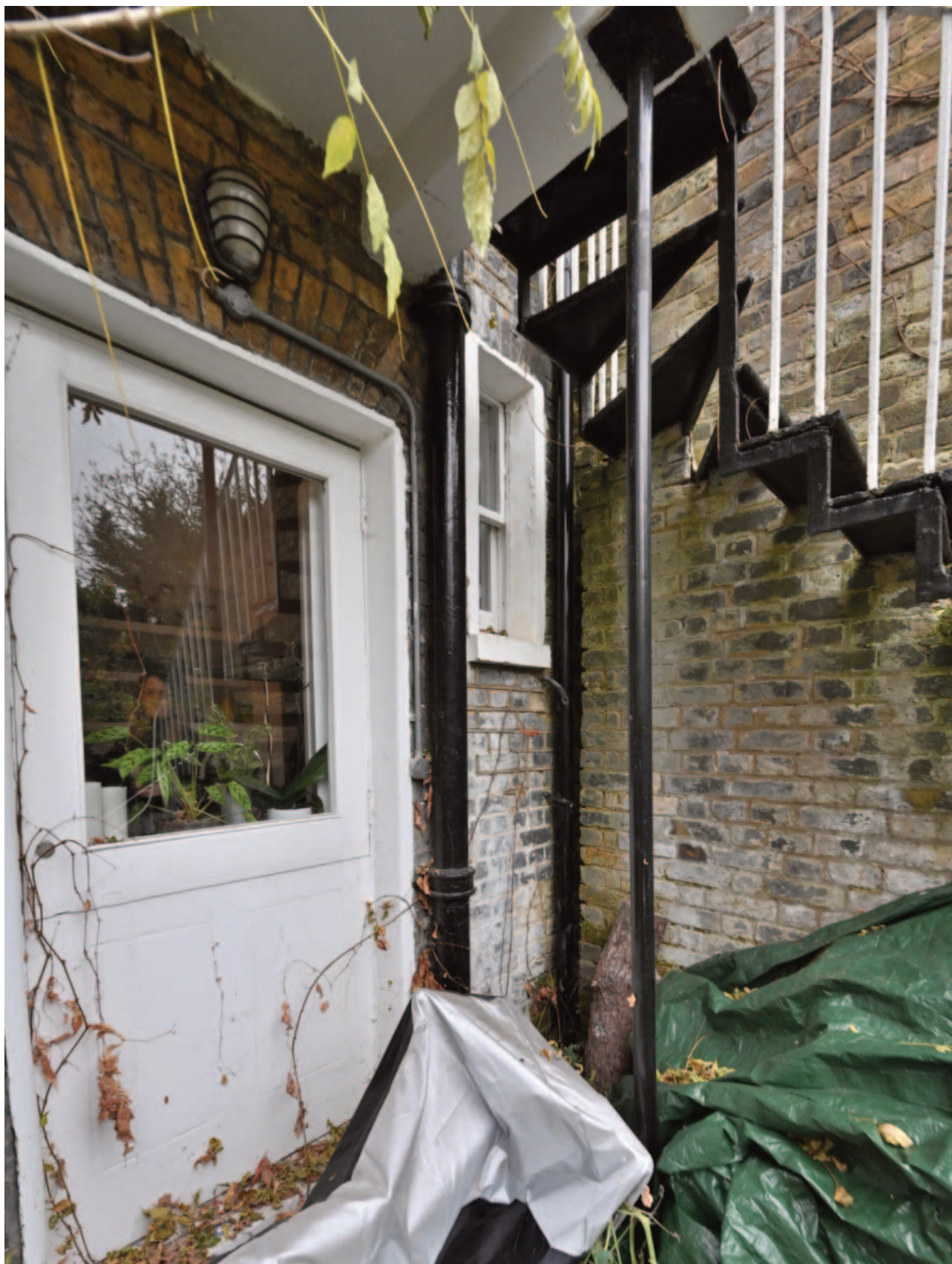
Fig. 16. The historic flush panelled door is inserted into an deepened former window (originally matching the window above), probably as part of the 1947 flat conversion because it has a slender wooden door-frame. It has subsequently been fixed shut and replaced above the lock rail by a modern side hung casement. In the foreground is a modern steel post supporting the replacement concrete balcony floor.
