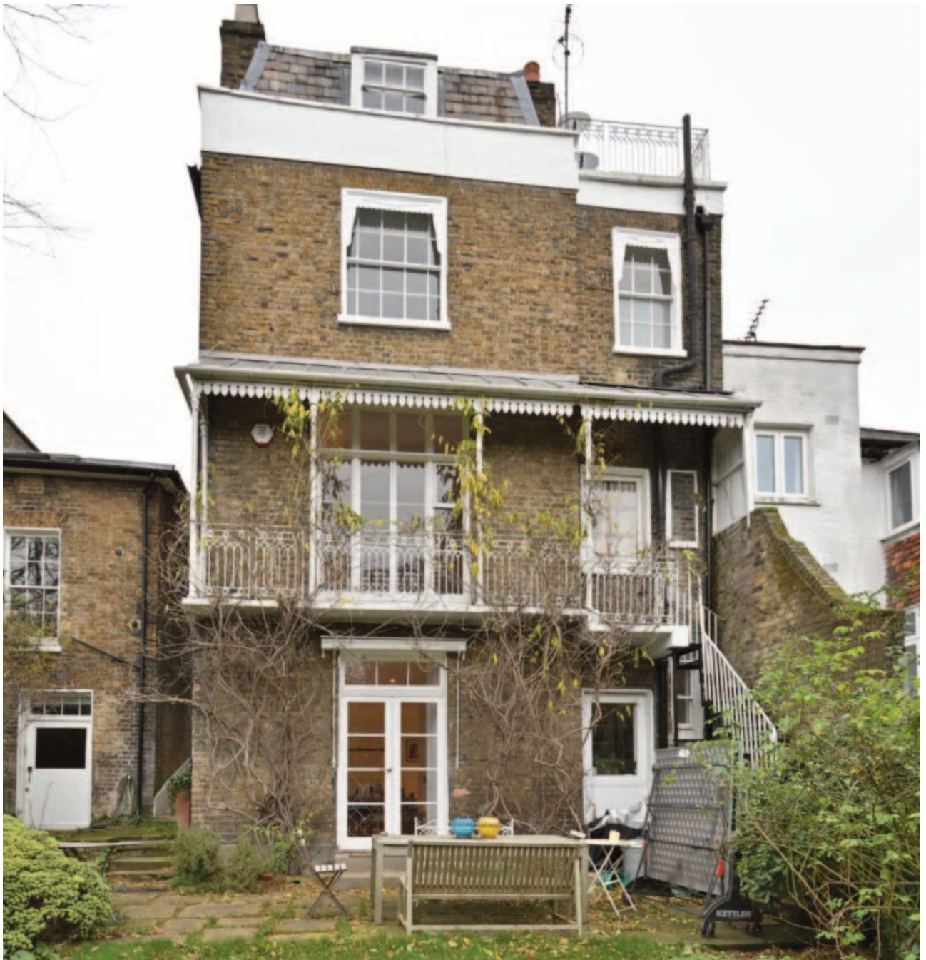
Fig. 15. The rear of the main house with inserted French doors replacing a sash window to the semi-basement floor and the partly rebuilt verandah with its cast concrete deck and replacement staircase and roof.
