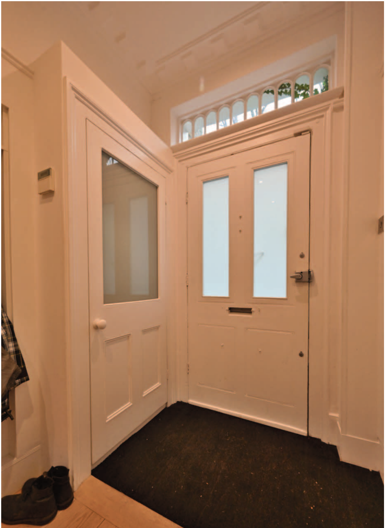
Fig. 21. Immediately adjacent to the front door is a modern cupboard containing services - perhaps reusing the architrave & door from the adjacent blocked doorway into the front room, which is now an open recess.
