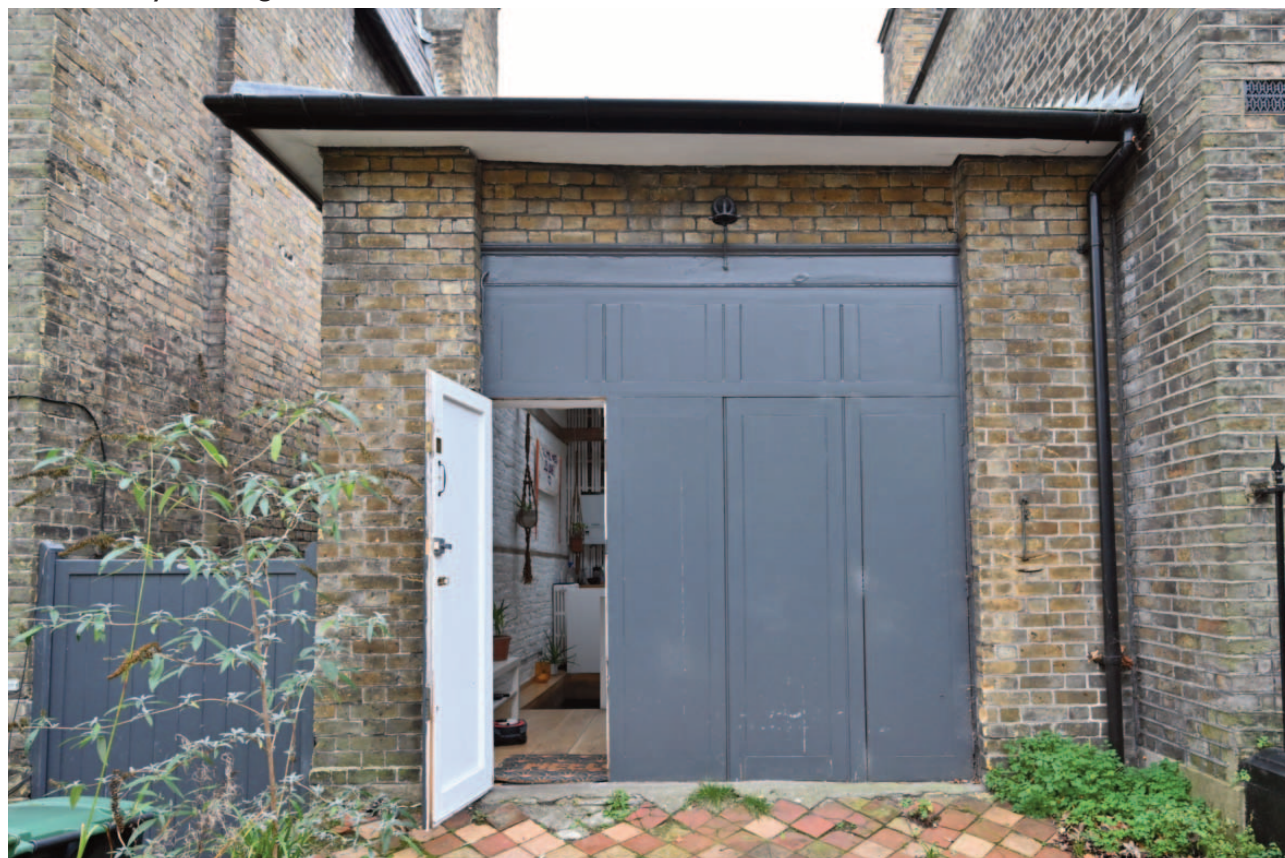
Fig. 11. The opening now reads as a four panelled folding door, but only the left hand door now opens and inside, the building has been converted to provide ancillary living accommodation on both floors.
