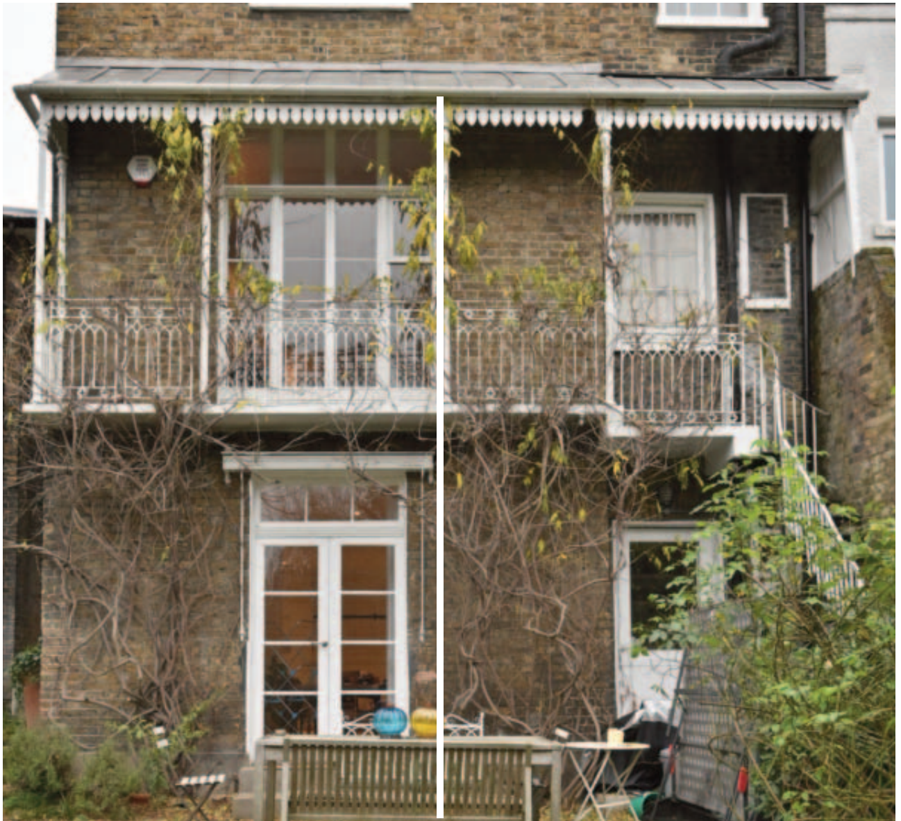
Fig. 17. The balcony retains its historic balustrade and decorative fluted cast iron posts and fretwork. The roof and deck are modern as is the additional corner post support adjacent to the stairs. Above the stair are the remains of a timber casement attached to the wall in front of a blocked window (which retains its flat brick arched head) matching the surviving window at semi-basement level below.
