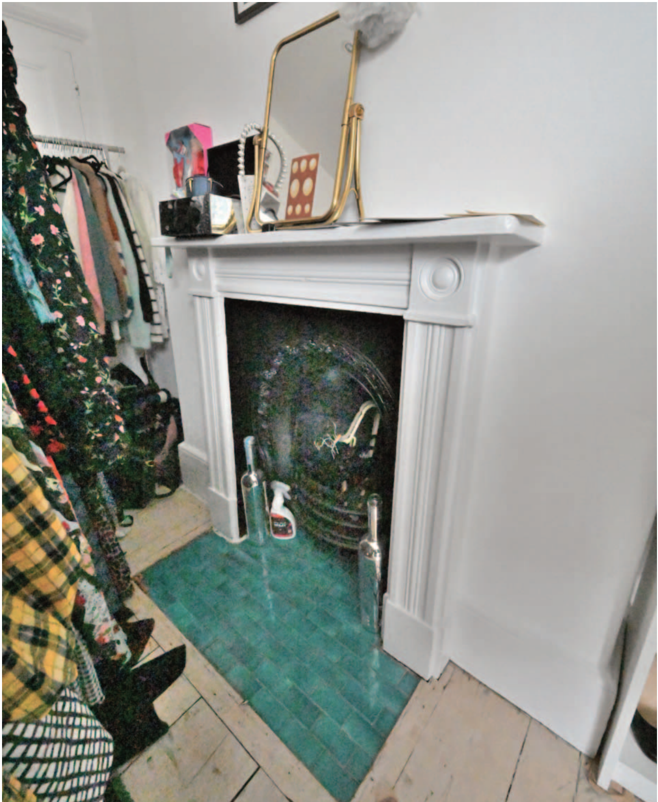
Fig. 38 The front bedroom in the main range with its mid 19th century detailing and later surround. Just visible behind is the door into the passage behind the attic stairs to the rear bedroom.
