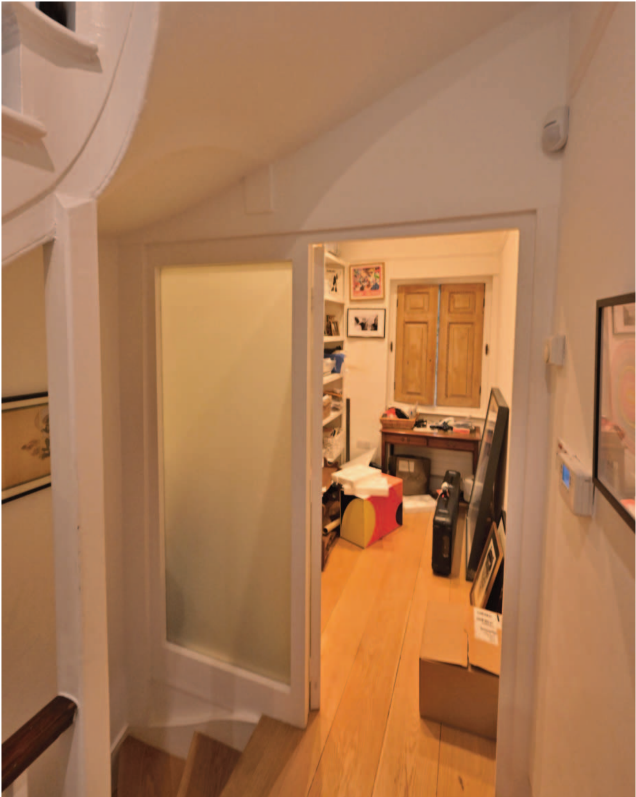
Fig. 22 The former historic W.C. and cloakroom at the south end of the east wing. The glass partition and door replaced a wall and door when the basement staircase was opened up. Only the shutters are historic.
