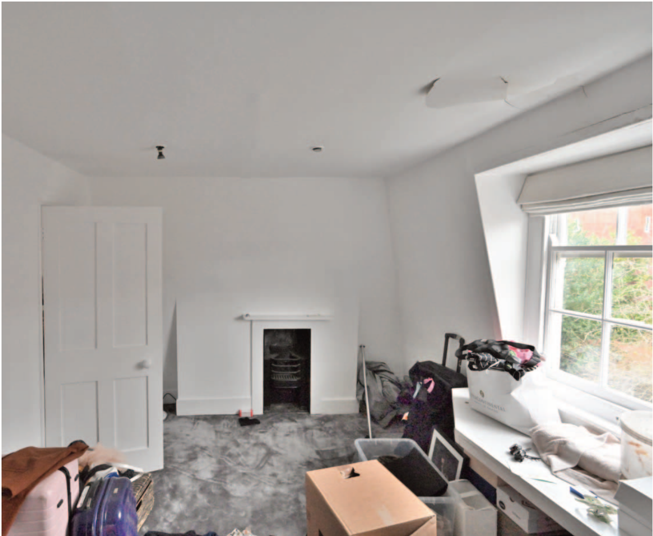
Fig. 41. The attic front bedroom with its steeply sloping walls and a small historic fireplace which appears to be in-situ . It is suggested that these attic rooms with their four panelled doors are of later 19th century date
