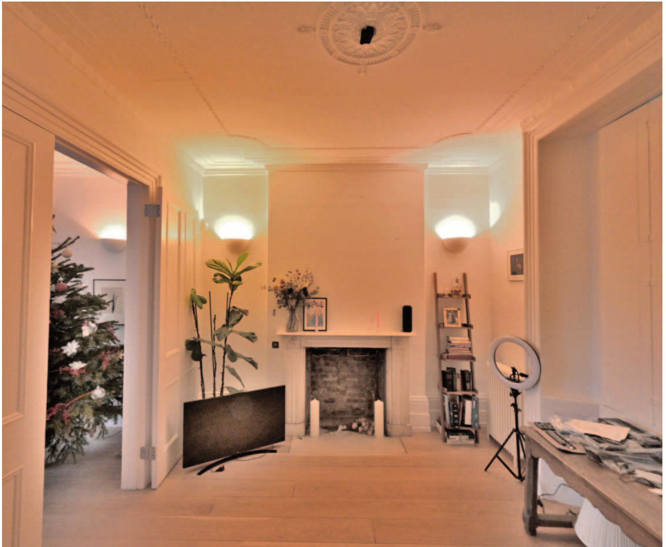
Fig. 26. The front room with its similar detailing including the deep stepped skirting, marble fire surround, ceiling rose and heavily overpainted cornice.
