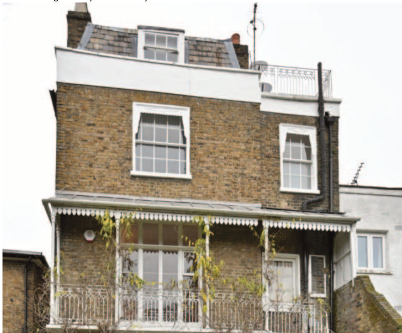
Fig. 18. The first floor windows retain their original external blind boxes and sashes. The attic windows are modern, and rendered has been partly rebuilt and the wrought iron balcony has been reset.
