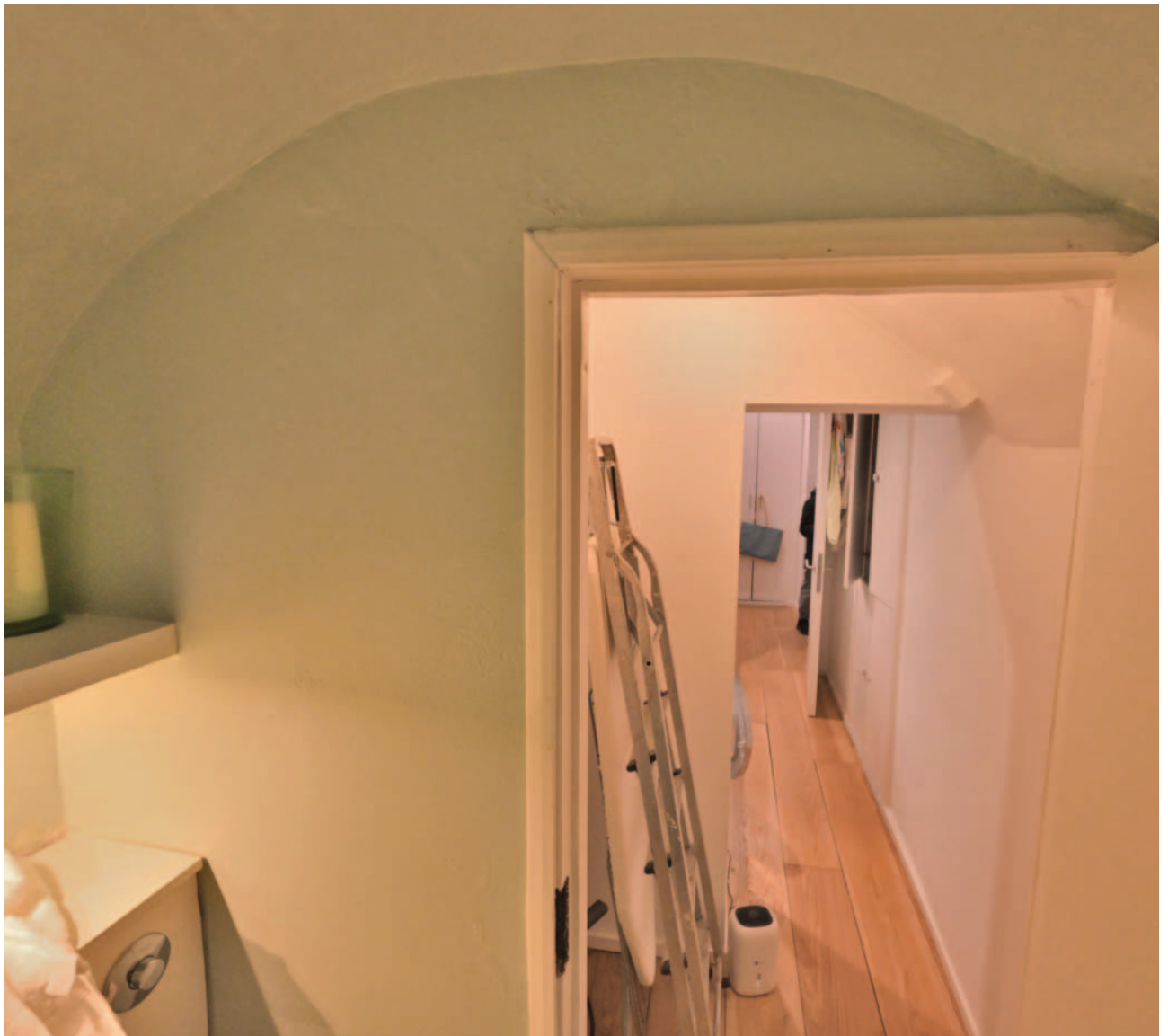
Fig. 30. The external vault below the front pavement is now a W.C. and utility area adjacent to the front basement room. A blocked door into this utility room is now a cupboard (visible on the right).
