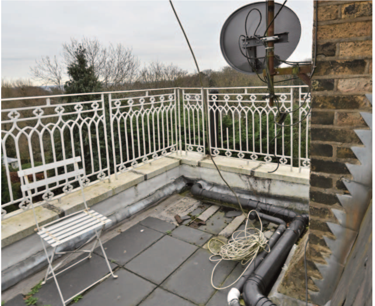
Fig. 19. The parapet to the flat roof of the east wing has been partly rebuilt in the later 20th century and the railings reset. The D-section handrail is a later alteration although the panels appear historic ones.
