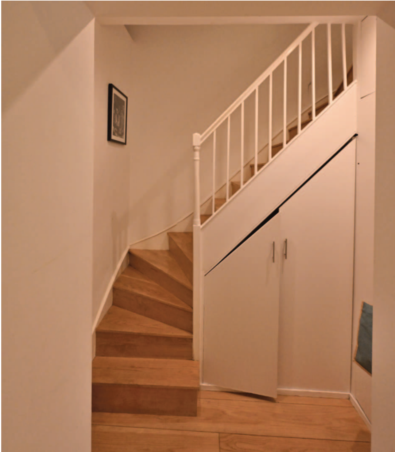
Fig. 29. The modified basement stair - note how the lower winders crash into the skirting and project beyond the newel post. The straight flight may be historic but the underside is concealed by modern finishes.
