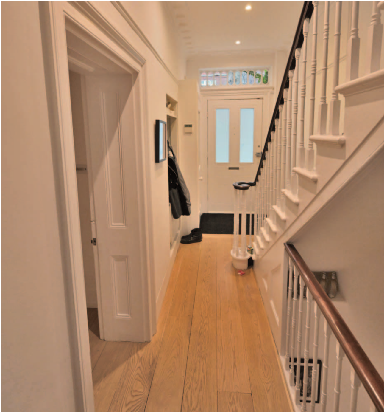
Fig. 28. The open basement stair with its modern balustrade replacing the original panelled infill, only a small area of which remains. Note the blocked doorway and inserted service cupboard by the front door
