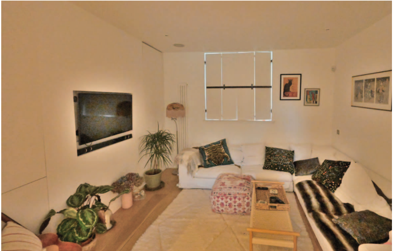
Fig. 32. The front basement room has a modern ceiling, wall and floor finishes and a television set into the former chimney breast. The door into the service passage on the right has been infilled.
