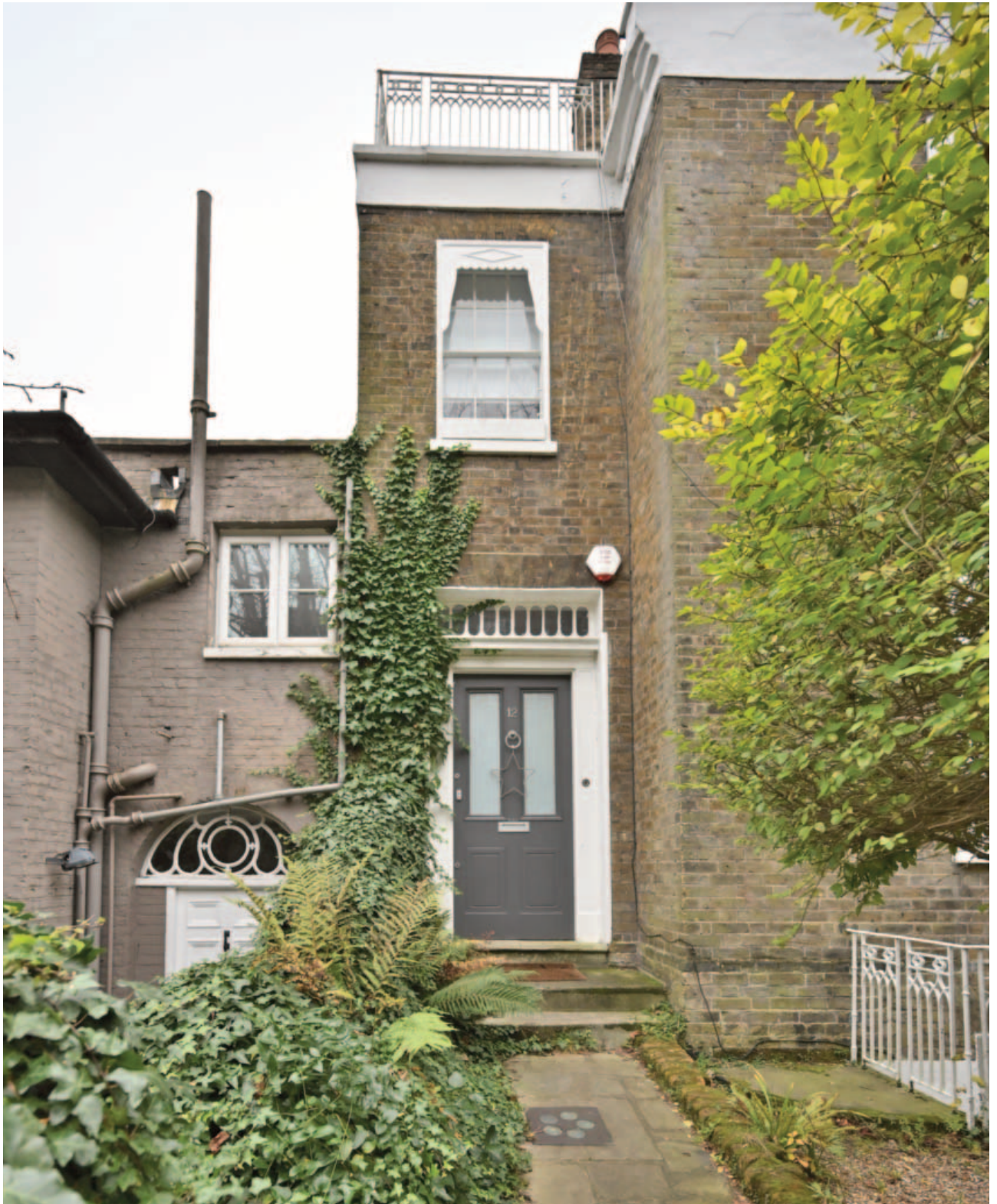
Fig. 8. The front door is located within the recessed side range. The flat roof to this range has 20th century railings matching those round the front lightwell. Its rendered eave cornice is also of 20th century date.
