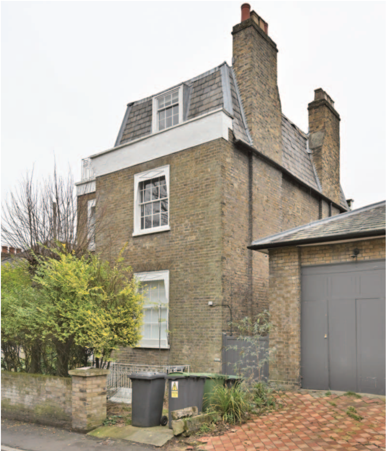
Fig. 7. The modern infill to the vaulted opening beneath the paved entrance way and the modern steep base-ment steps and railing detract from the fine quality of the principal elevation.
