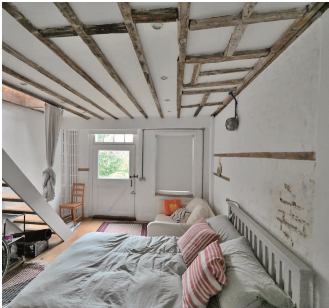
Fig. 46. The basement room - originally a stable it was converted to a workshop by the addition of a hearth to the left and a window to the right of the door. The stairs are modern and not in their historic position.
