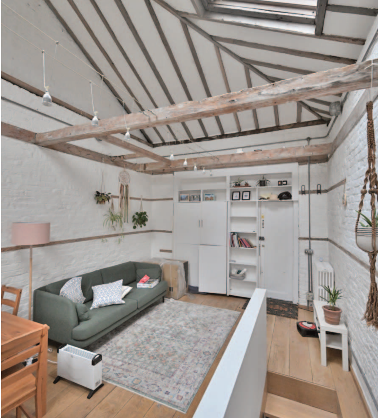
Fig. 45. The front of the upper floor showing cupboards built on the inside of the historic door opening from the lane. The ceiling structure suggests there was originally ladder access up to storage within the roof.
