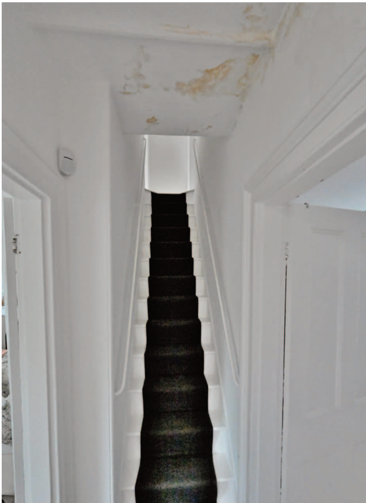
Fig. 38. The small lobby at the foot of the narrow attic stairs opens into the principal bedroom on the south (rear) whilst a similarly detailed door opposite opens into the smaller front room.
