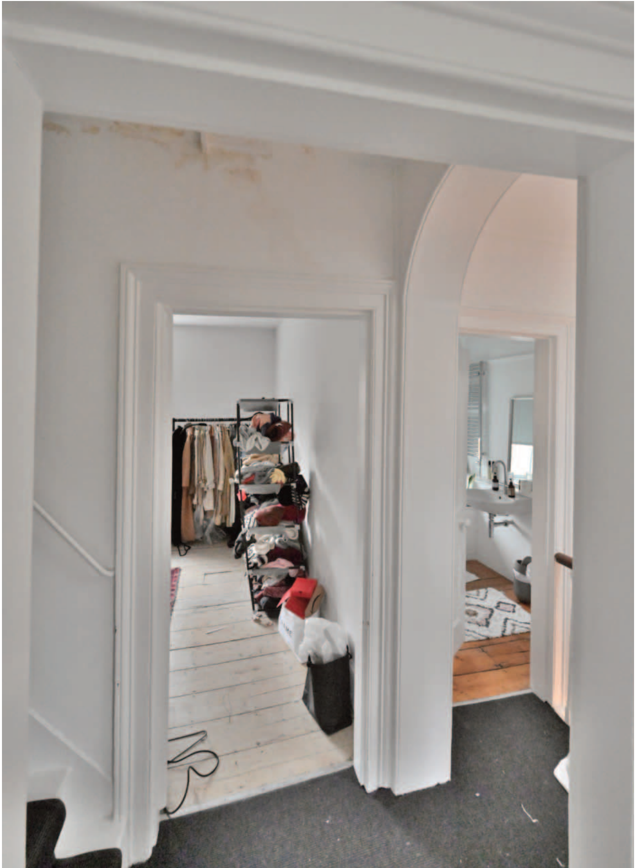
Fig. 35. Detail of the small lobby at the foot of the attic stairs with the arched opening from the stair hall. The architraves and doors share the same detailing although the cornicing is simpler at this level.
