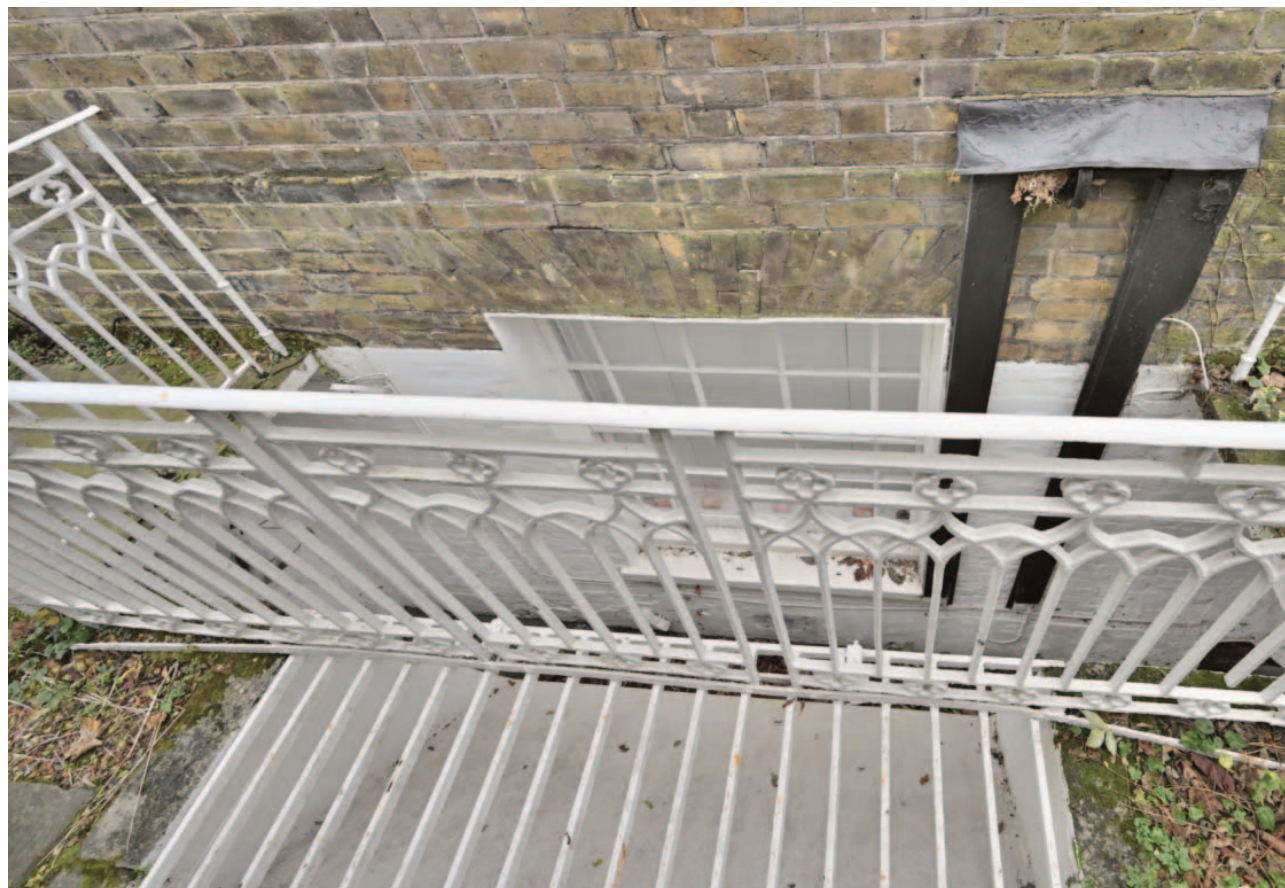
Fig. 9. The front basement window with its narrower outer panes detailed to resemble margin lights. On the right are the remains of a 19th century service hoist on the right. The historic railings round the lightwell, (including an opening gate panel with a pivot) have been reset beneath a later D section handrail.
