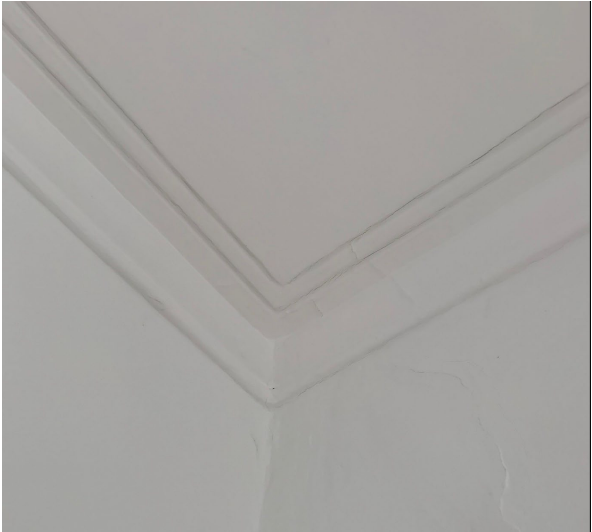
Fig.05 – Survey photo taken in 2022 for other proposals showing the original cornice to be copied including inset detailing.
