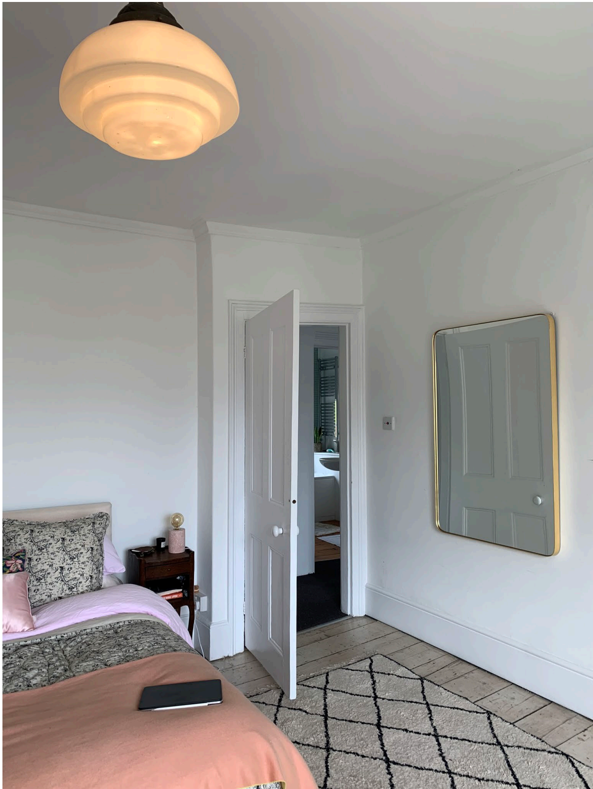
Fig.06 – Survey photo taken in 2022 showing the original cornice to be copied.
