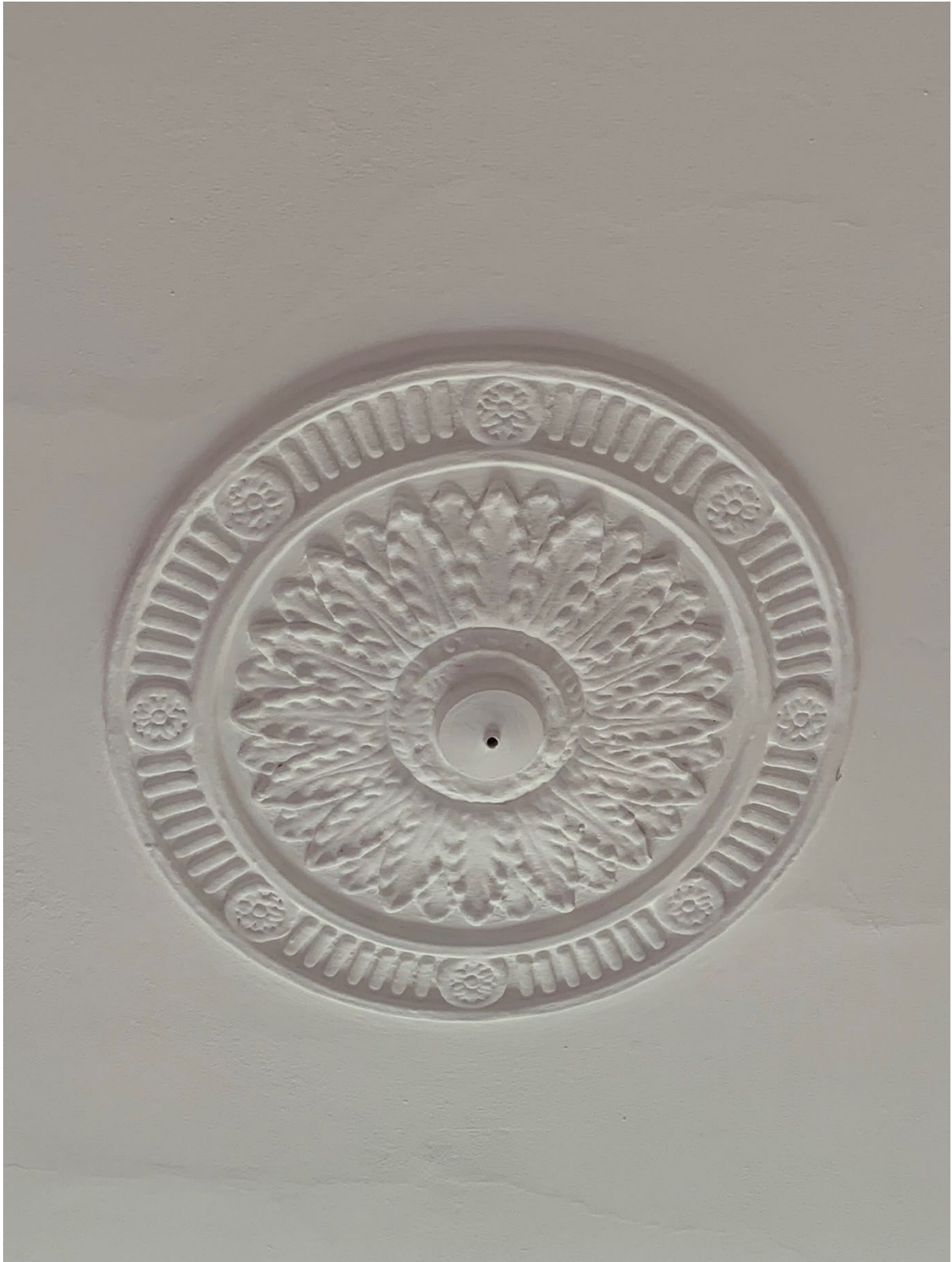
Fig.07 – Pre-flood damage house survey photograph showing modern ceiling rose. Although not original and adhered to the lining paper this is to be replaced to match existing.
