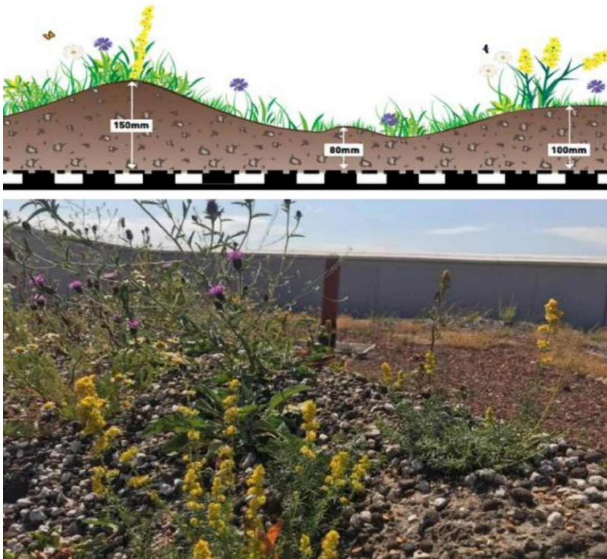
Figure 5.1 Example substrate type and planting variation on biodiverse roofs (please note depths shown are not those specified for this site)
