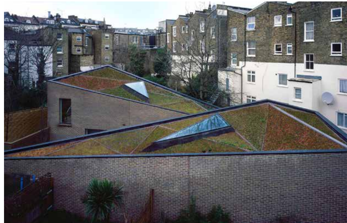
VPPR; Angled green roof forms with triangular skylights
