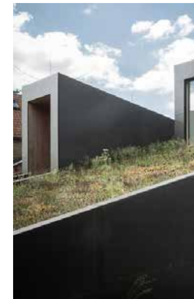
Angled green roofs
