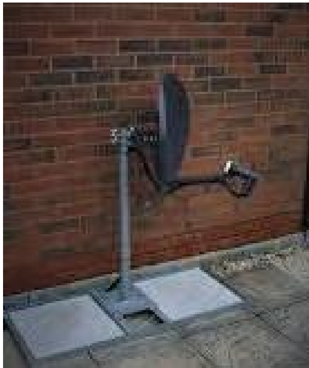
Dish mounted on 600mm pole fixed to roof
