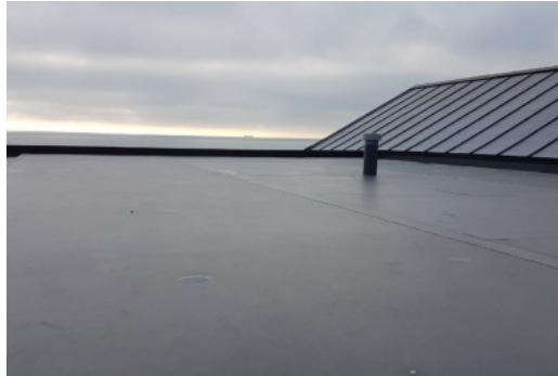
Renolit Single PLY Membrane- salmonsolutions.co.uk
