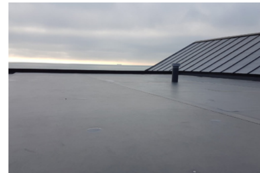
Renolit Single PLY Membrane- salmonsolutions.co.uk
