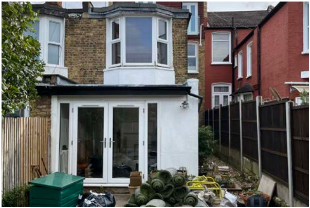
External rear view of existing
