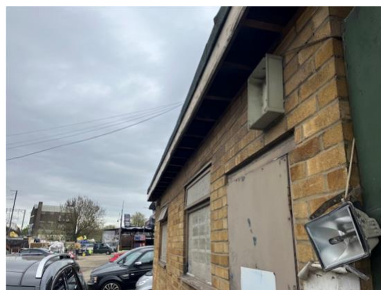
Photo 7: exposed roof beams at end of building.
