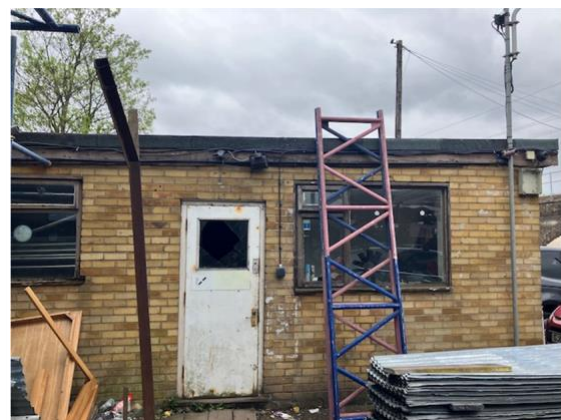
Photo 6: building on site showing flat roof and intact windows and door.
