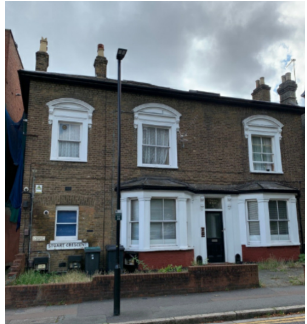
Existing building at 4 Stuart Crescent
