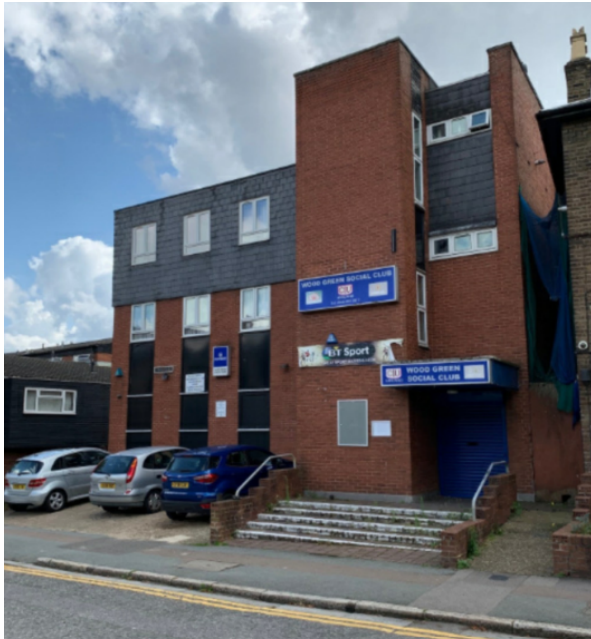
Existing building at 3 Stuart Crescent
