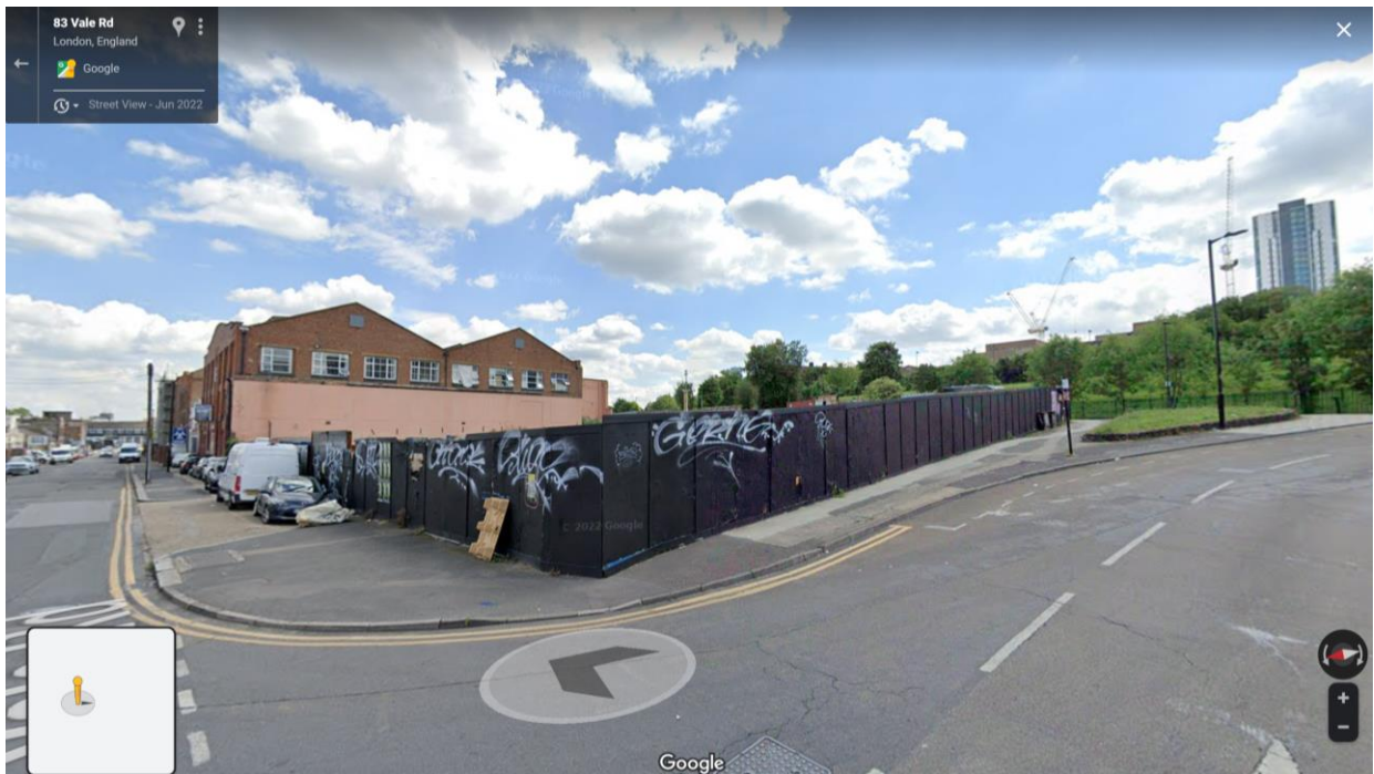
View of site from Linkway.
