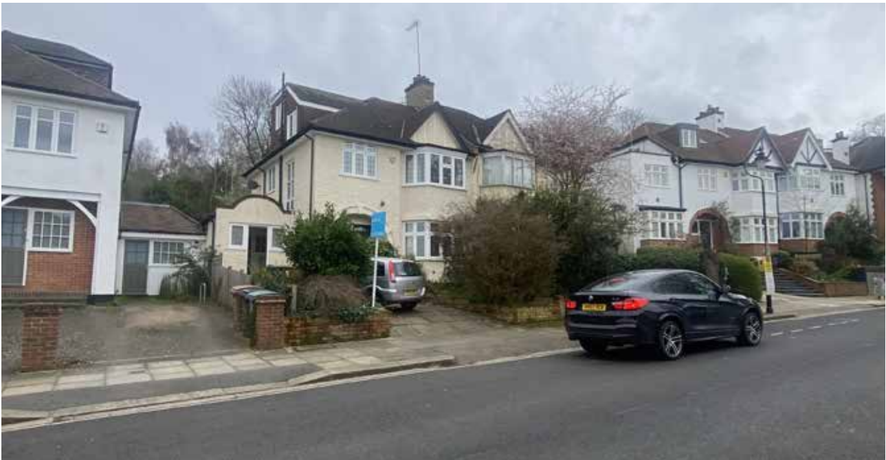
[Fig. 01] View of street facing facade of 13 Cholmeley Crescent
