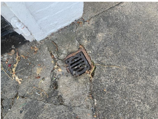
Drainage grate located adjacent to front gate.
