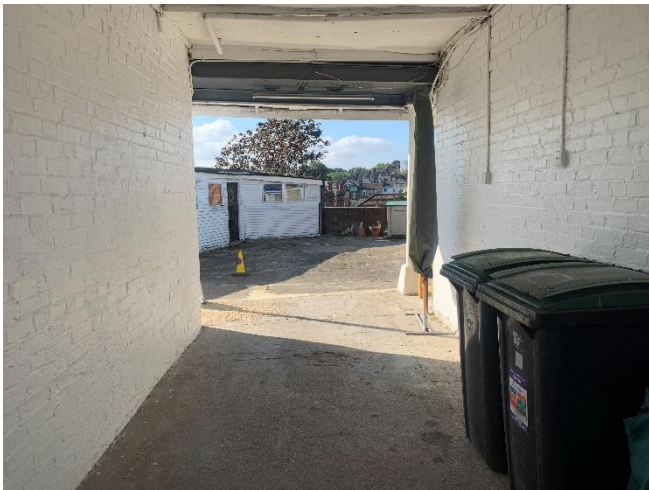
S facing view of entrance passage leading to rear courtyard
