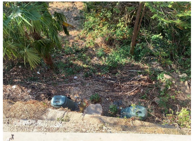
View of the estimated 8m drop adjacent to the southern side boundary.
