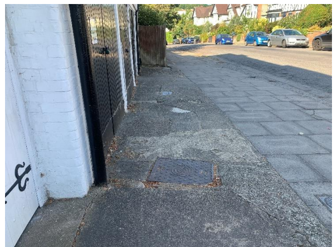
Manhole cover and drainage grates located along the northern site boundary.
