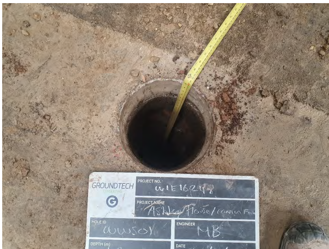
Photograph 4 – Concrete coring and hand pit of WWS01.
