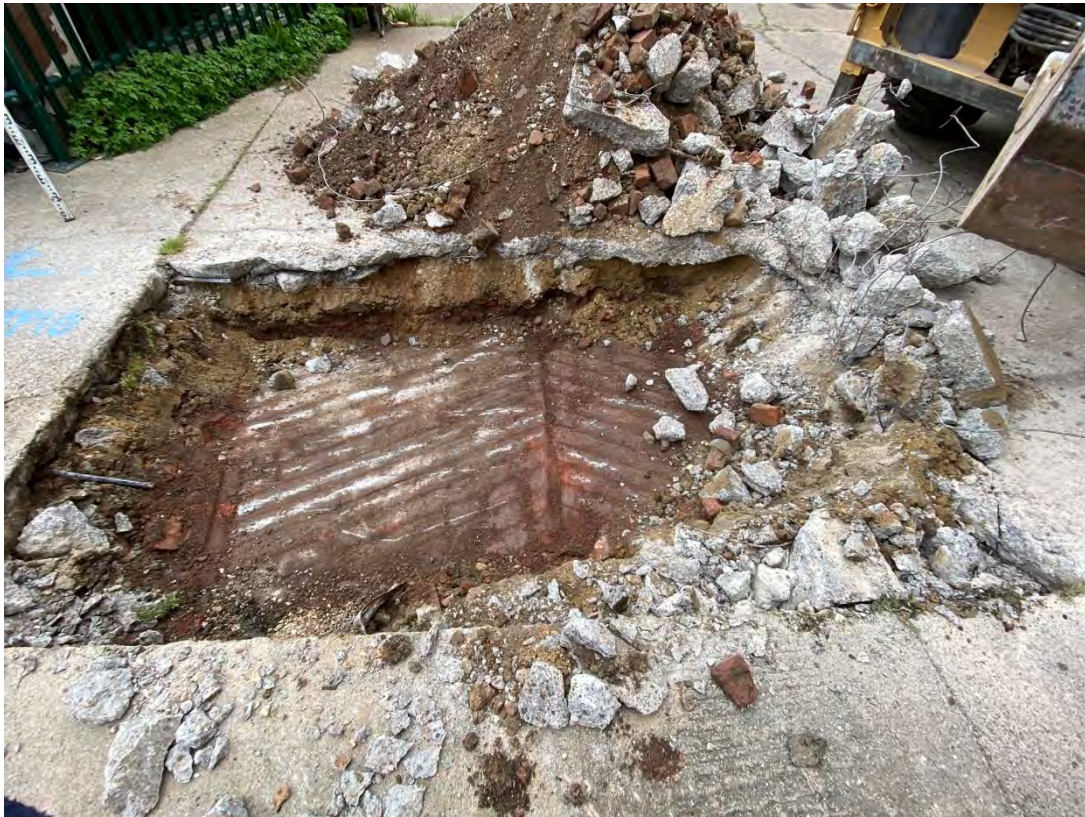
Photograph 13 – Concrete obstruction in WTP10 near underground tank.
