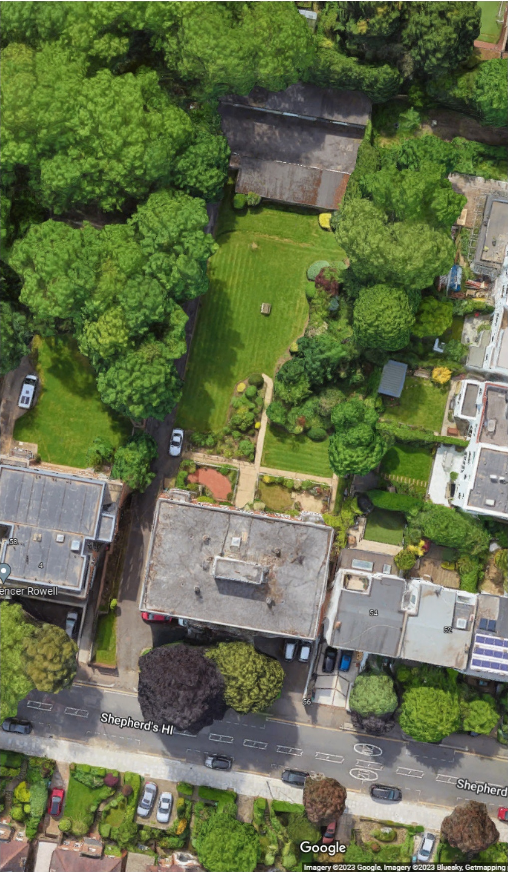
Aerial View of Site Before Demolition
