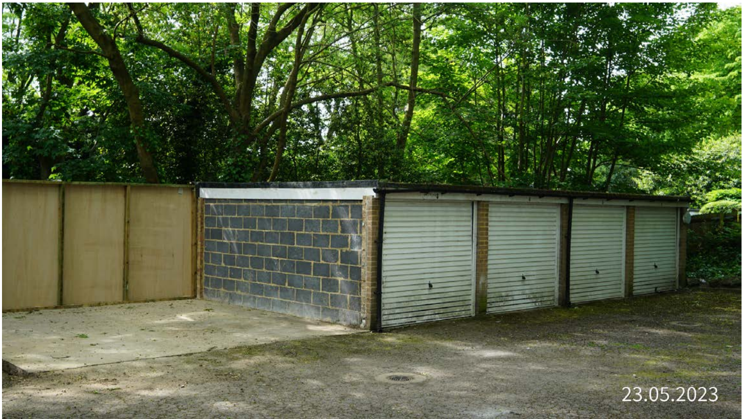
The photos above were taken during a visit to the site on the 23rd May 2023 following complete demolition of garages 1 & 2. A newly erected temporary hoarding along the rear boundary, can be seen, in place of the demolished rear garage walls. Garages 3, 4, 5 and 6 in this row, remain.
