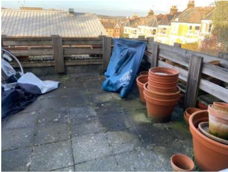
1. Photo looking north standing on roof terrace
