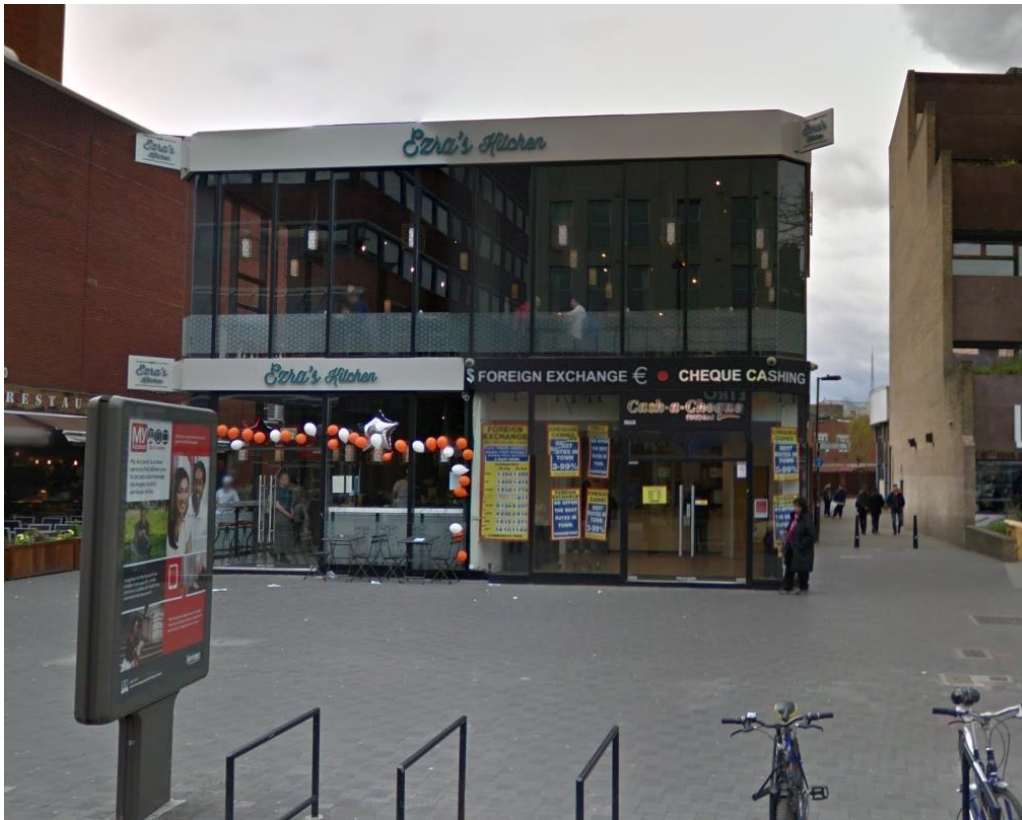
Pic.1 185 High Road, Front elevation
