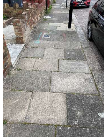
Photo 30 Partially damaged private wall
