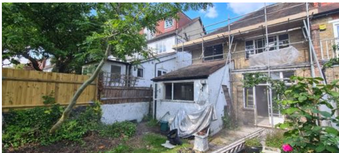
5. Rear view of 181 and 183 Park Road
