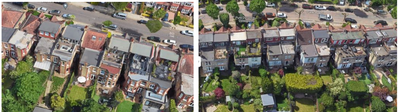
6. Examples of roof terraces on Park Avenue South and Farrer Road
