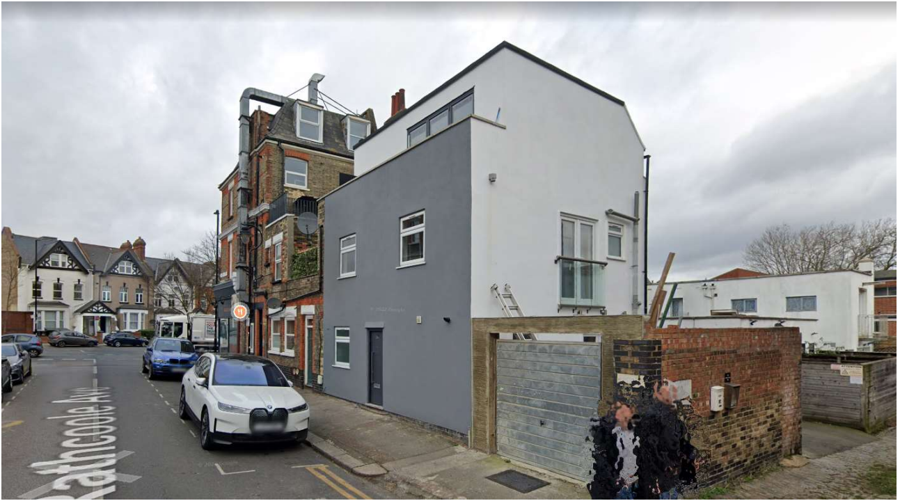
Existing street view
