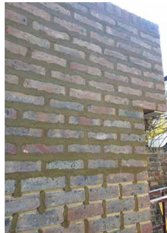
Pointing process - joints are raked and mortar applied to be flush to face of brick
