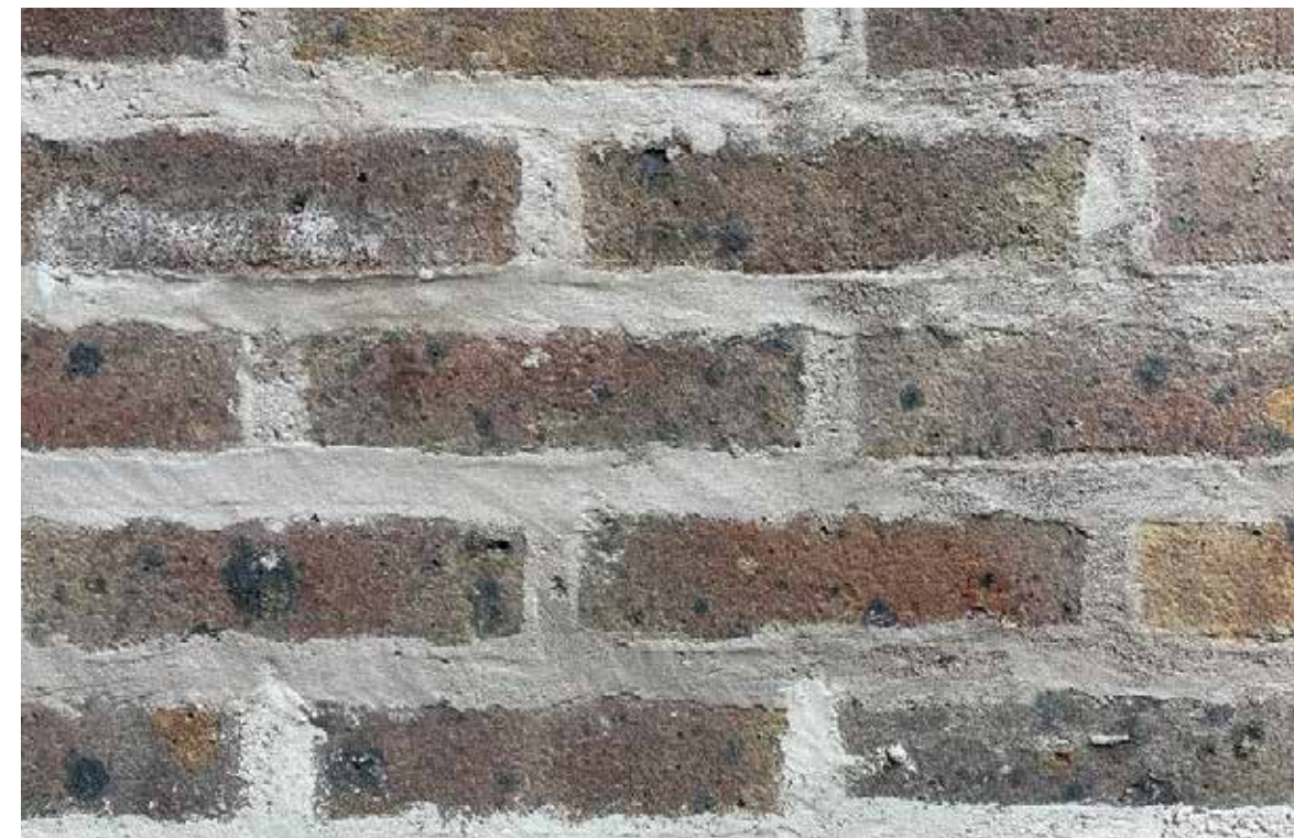
Sample prepared on site to show pointing - Selected Dark brick with Lime mortar
