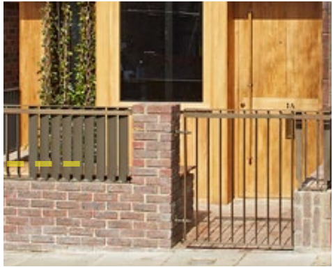
Front garden rails and gate
