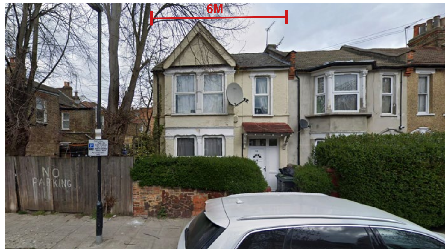
2. View looking towards 48 Argyle Road
