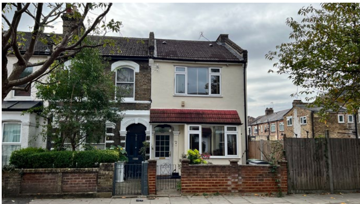
3. View looking towards 49 Argyle Road
