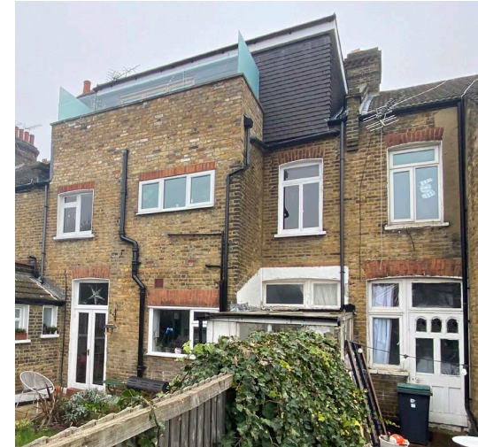
19 Whitley Road - neighbouring terrace and dormer extension
