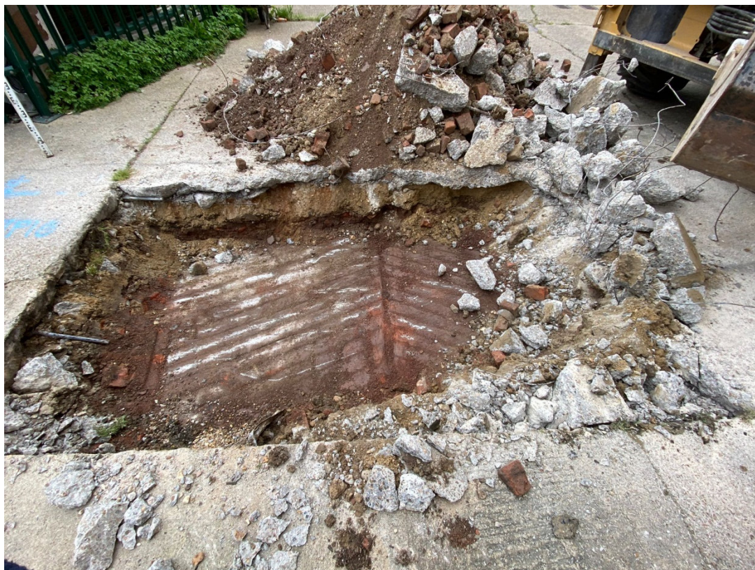
Photograph 13 – Concrete obstruction in WTP10 near underground tank.
