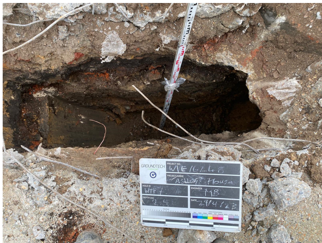
Photograph 13 – Concrete obstruction in WTP10 near underground tank.
