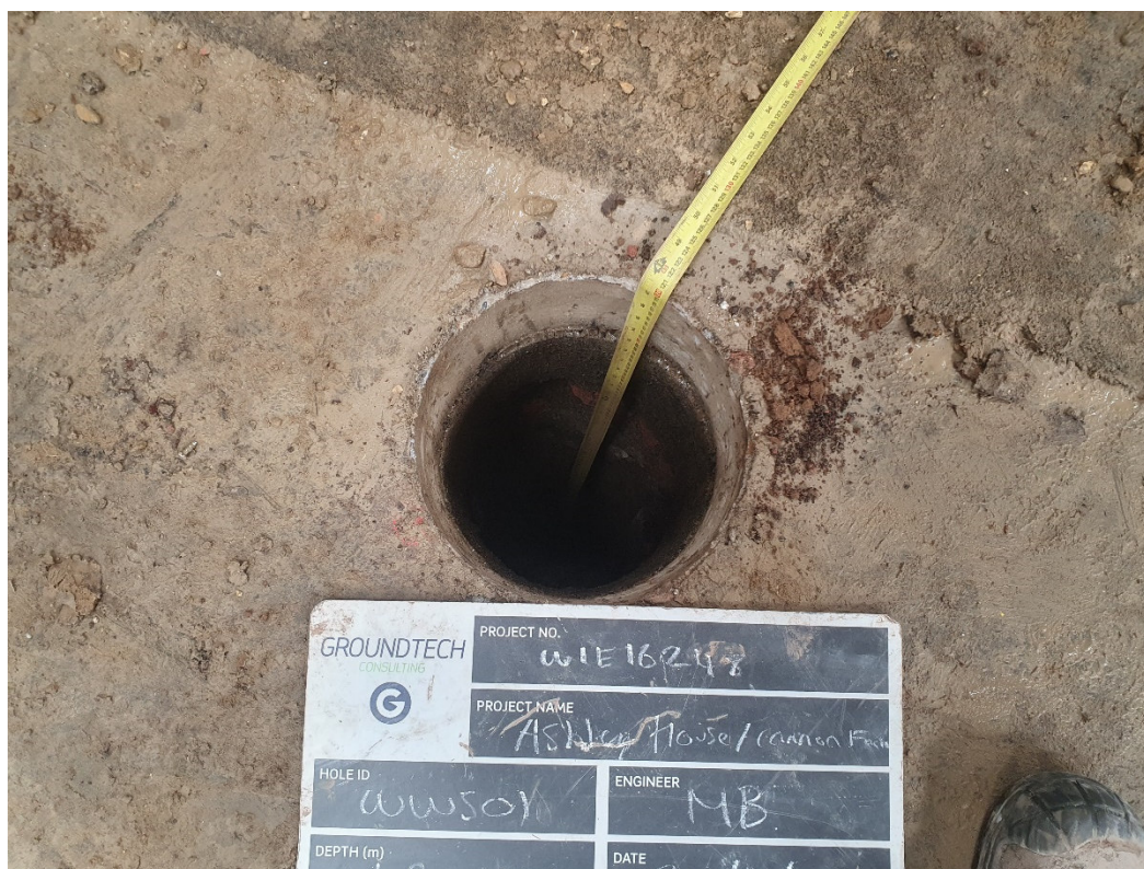
Photograph 4 – Concrete coring and hand pit of WWS01.
