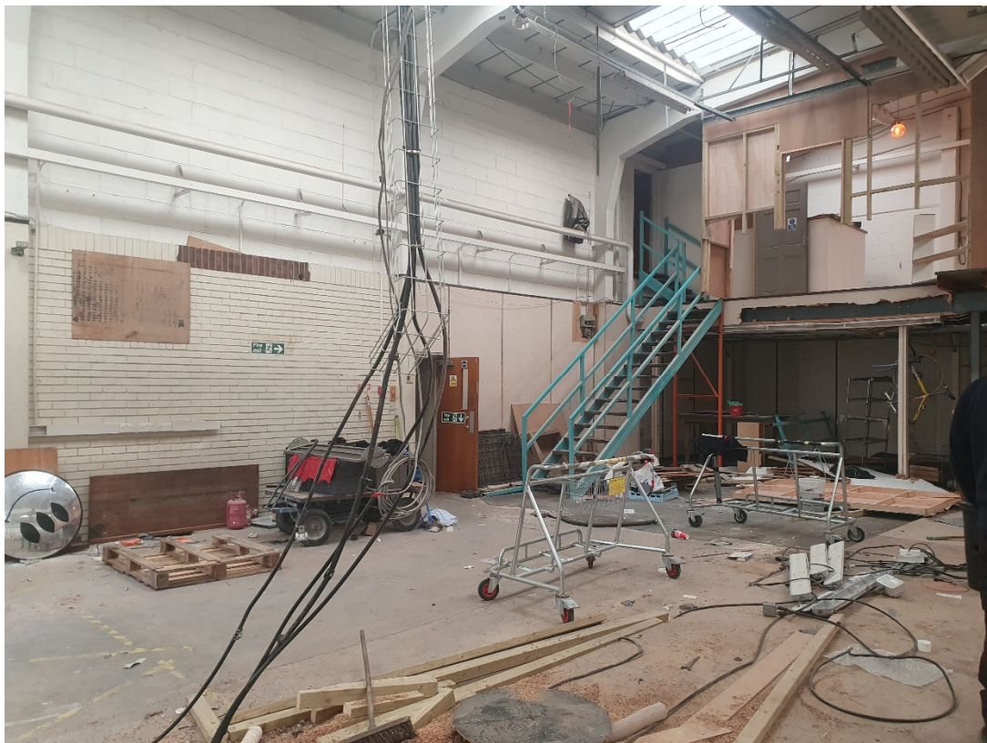
Photograph 1 – Internal area of Cannon Factory looking towards WWS01.
