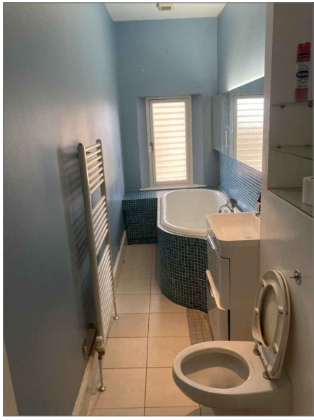
BATHROOM TO BE ALTERED
