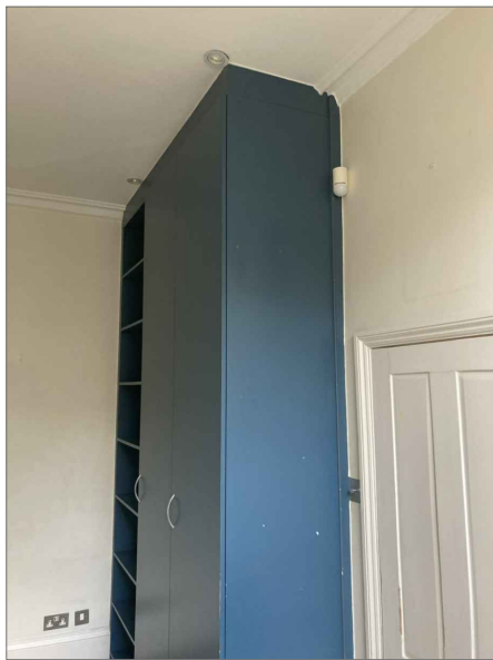
CUPBOARD TO BE REMOVED
