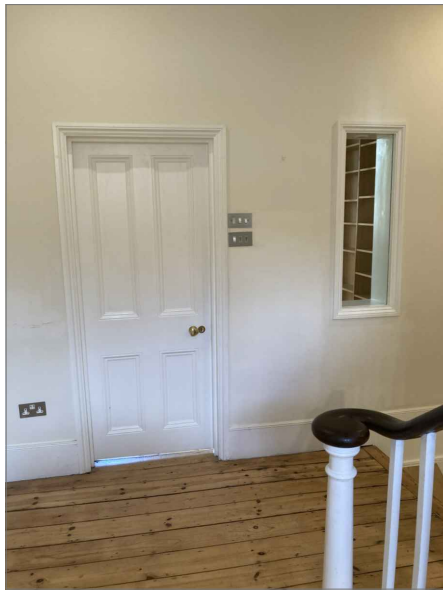
OPENING TO BE INFILLED
