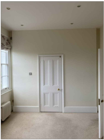
SHOWER ROOM TO BE DEMOLISHED
