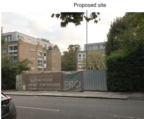
View of the proposed site from Stanhope Road
