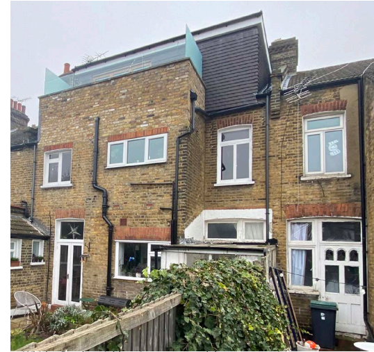
19 Whitley Road - neighbouring terrace and dormer extension
