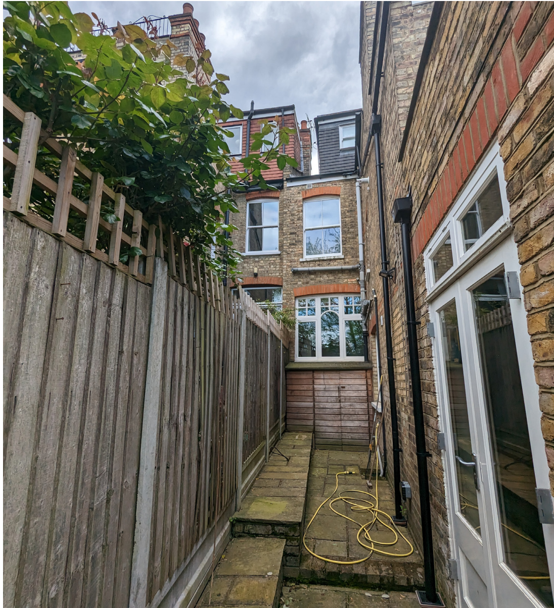
View down side of outrigger towards main house
