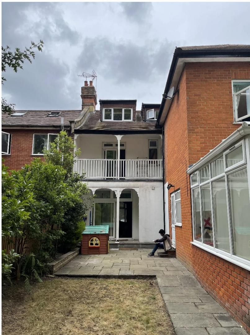
Pic 2: 12 Colney Hatch Lane – Rear view
