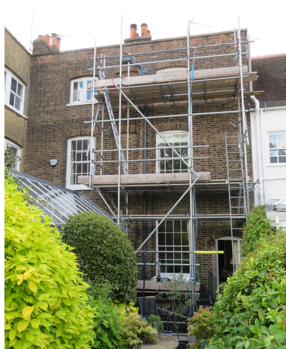
Rear elevations of 47 and 49 North Road. Note the blind window on the party wall line.
