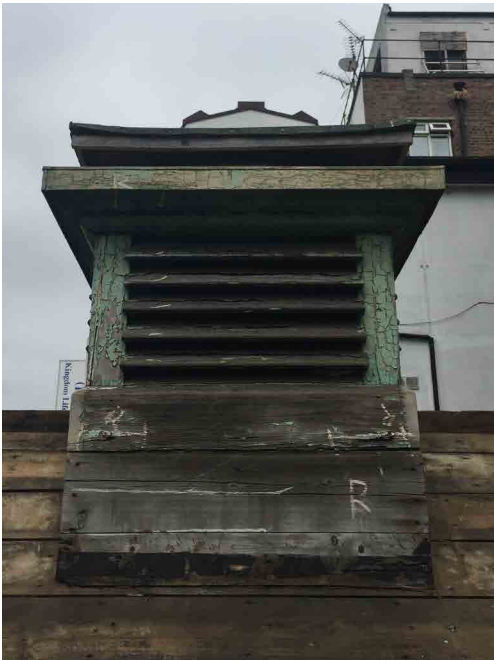
5.1 South-east elevation Timber mostly in sound condition, small localised repairs marked Paint removal commenced, to be repaired and redecorated in line with method statements
