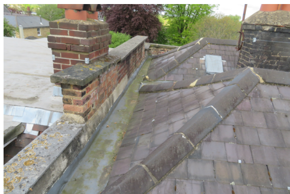
The hipped ends of the front and rear roofs, looking west.
