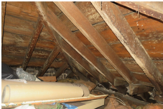
Interior of the front roof looking to the south east.
