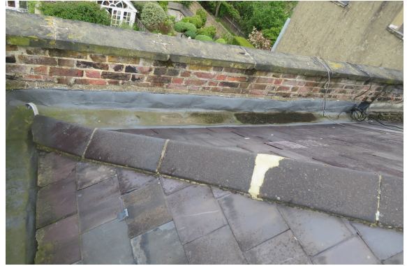
Rear parapet gutter.
