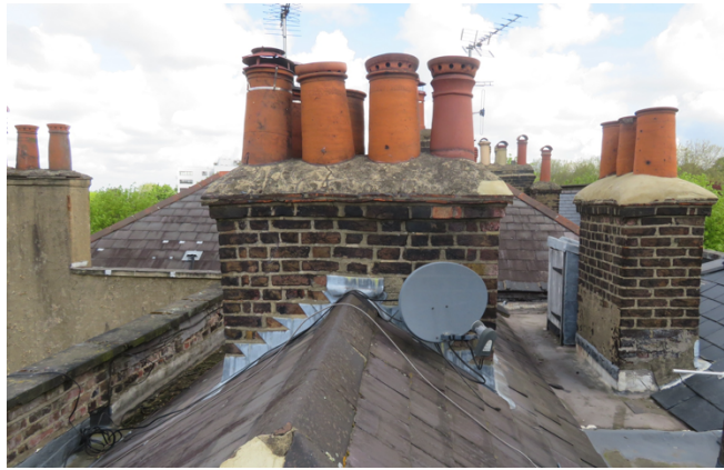
The large chimney stack to the rear roof.
