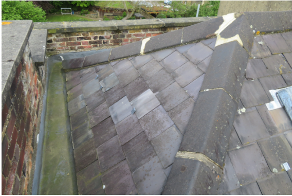
Southern hip to the rear roof looking west. Note York stone parapet copings, mortar infill to the hip tiles and slates held on clips.
