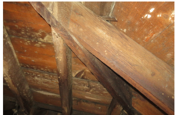
Some of the roof timbers appear to be of oak.
