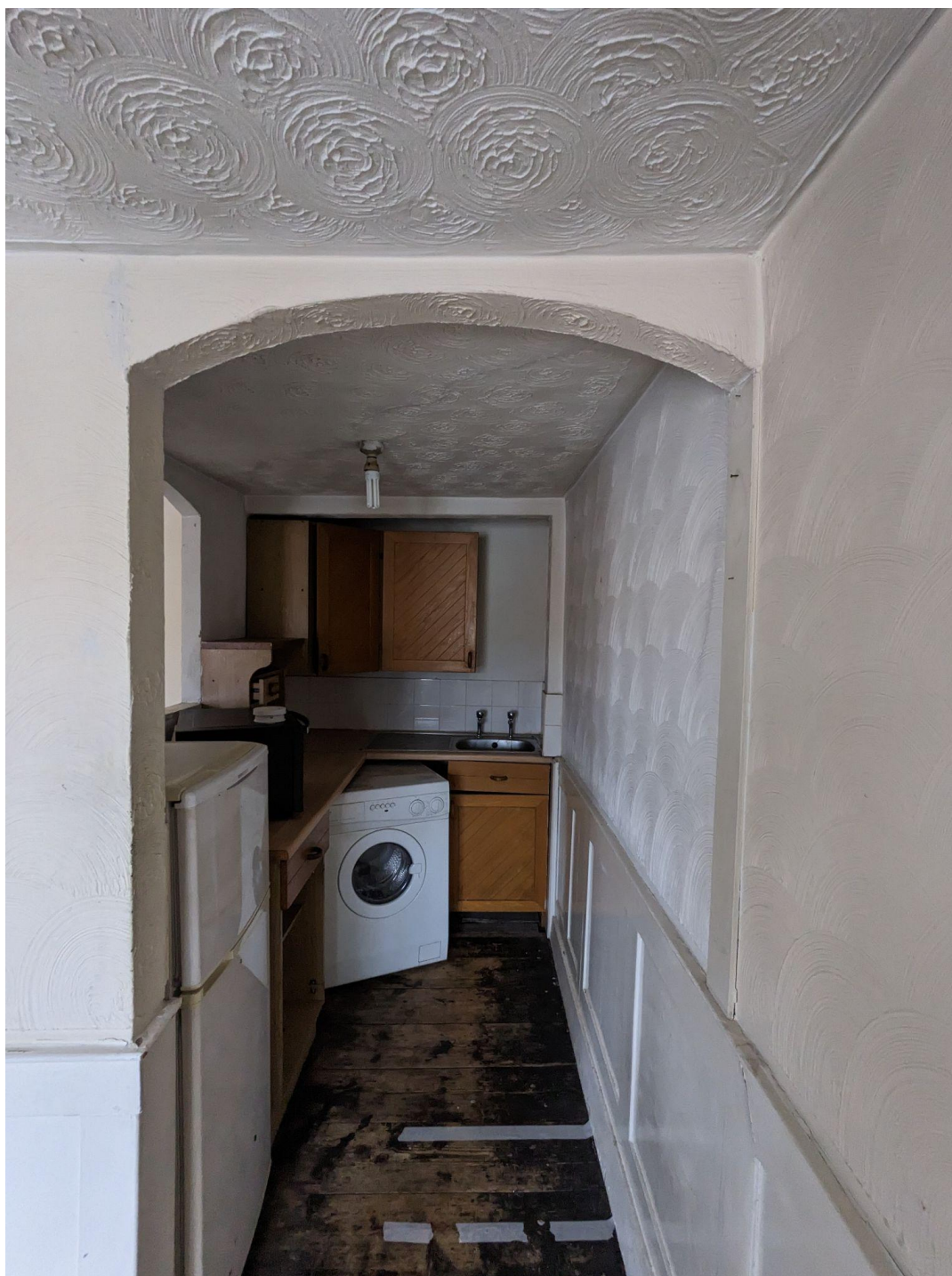
Internal view of wall proposed to be removed 2
