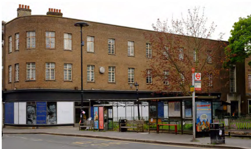
23A Front elevation of the Broadway Annexe, west block (2017)
