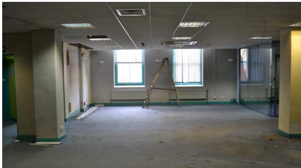
33 Interior of east block of the Broadway Annexe (former telephone exchange), 2017
