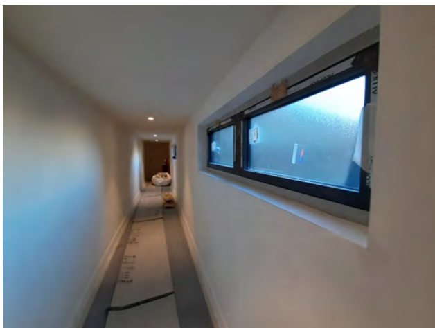
31E Broadway Annexe first floor corridor west block
