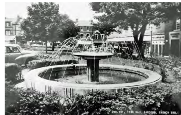
10F Forecourt and fountain, c. 1960s (Haringey Archives)
