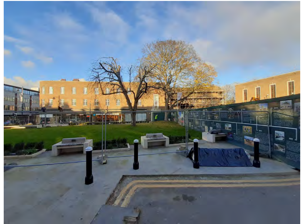
21A Broadway Annexe south elevation, showing the east (R) and west blocks (L)
