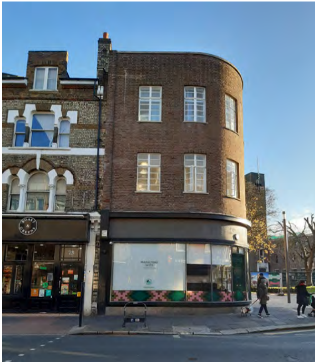
22 Broadway Annexe west elevation facing The Broadway
