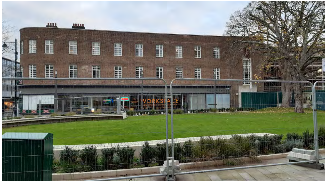
23 Broadway Annexe south elevation, west block
