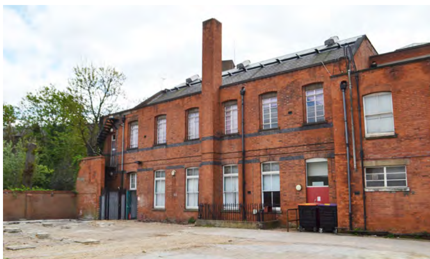
24A Rear elevation of the Broadway Annexe, east block (former telephone exchange) (2017)
