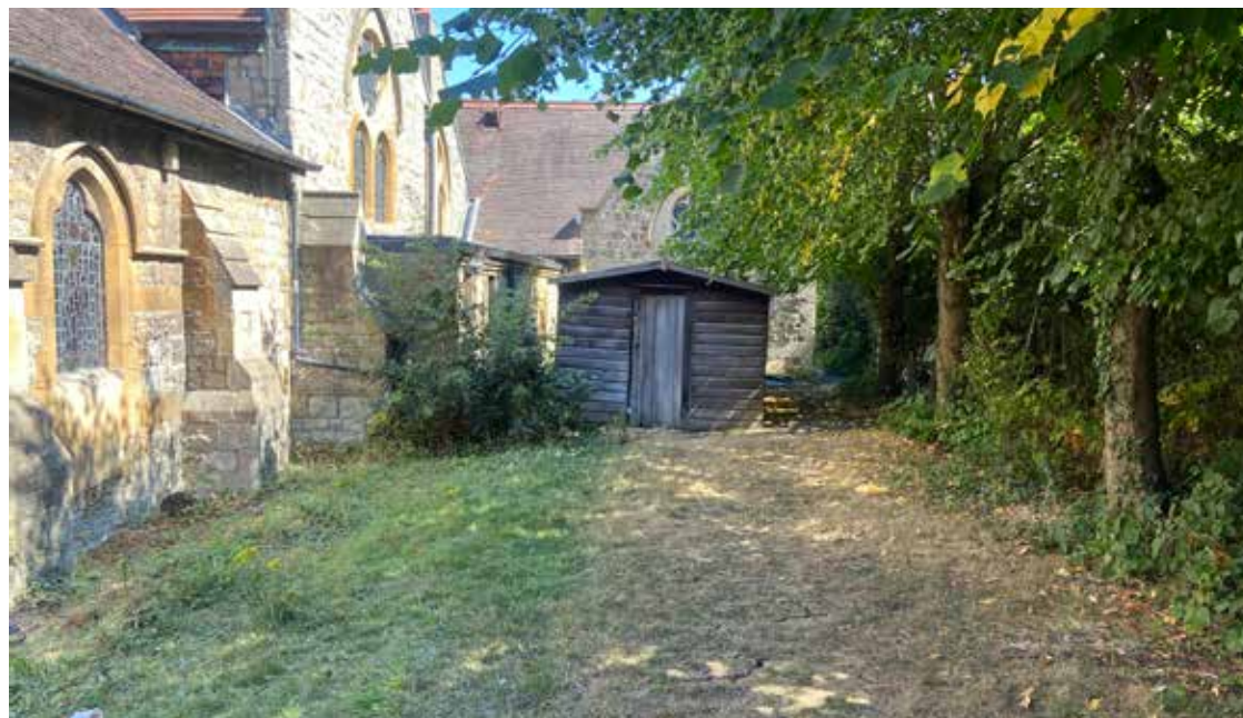
The existing shed
