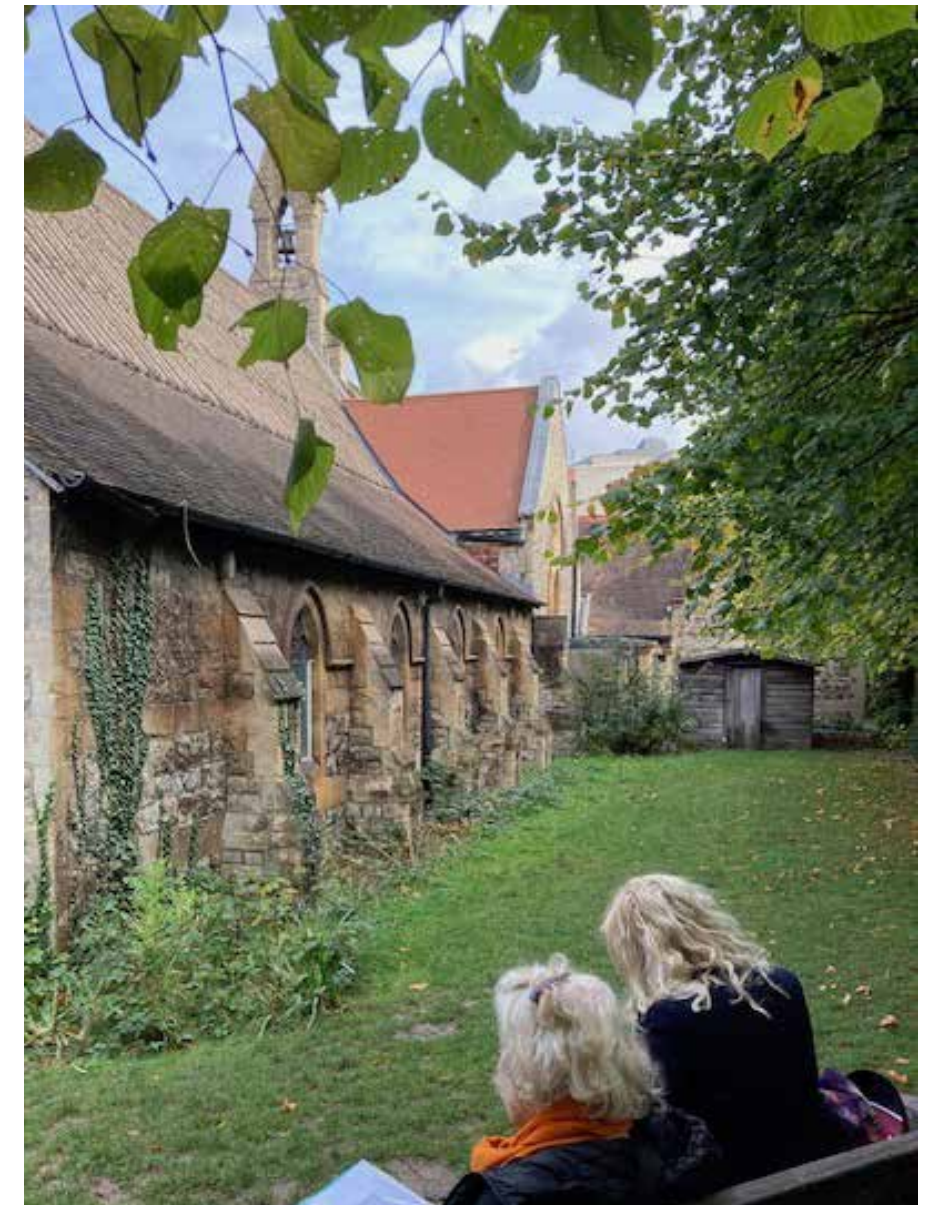
View along the south side of the Church towards the existing shed
