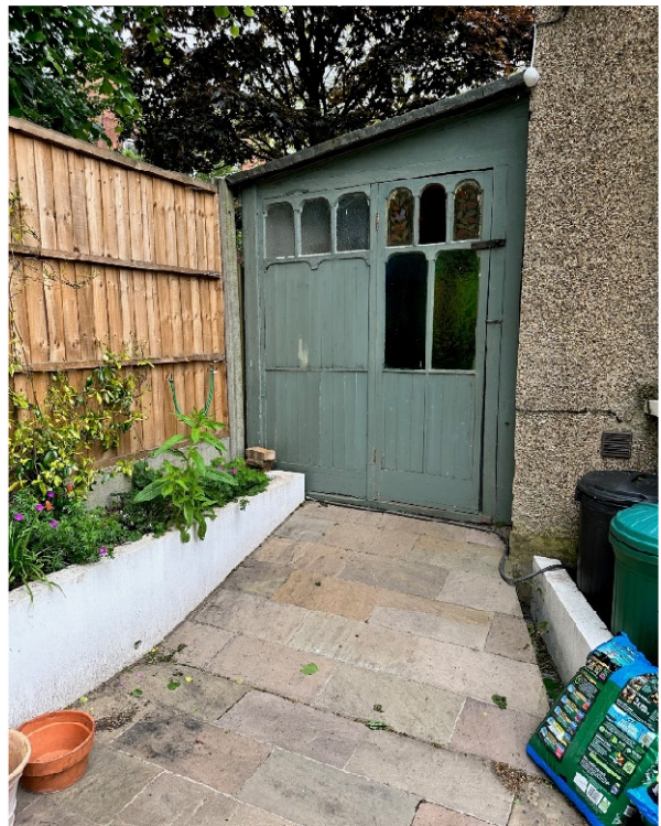
Shed to be demolished.
