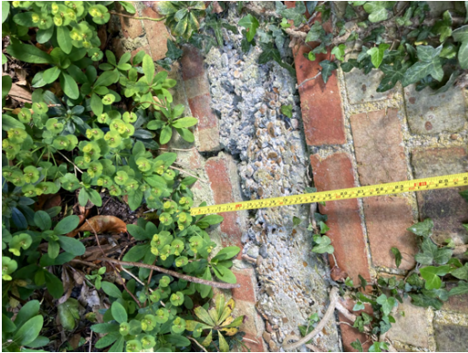
10. Base of boundary wall to 11 - 14 Highbank Way
