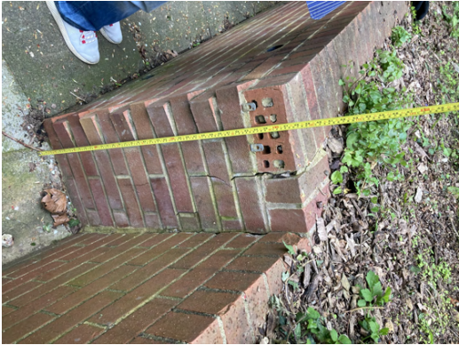
7. Existing brick retaining wall to Highbank Way Alleyway
