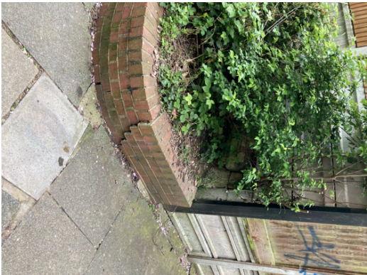
5. Existing brick retaining wall
