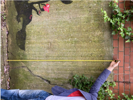
4. Retaining wall of No. 14 Highbank Way Alleyway
