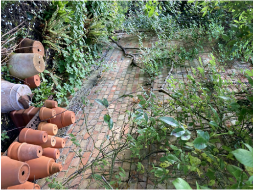
9. Boundary wall to 11 - 14 Highbank Way
