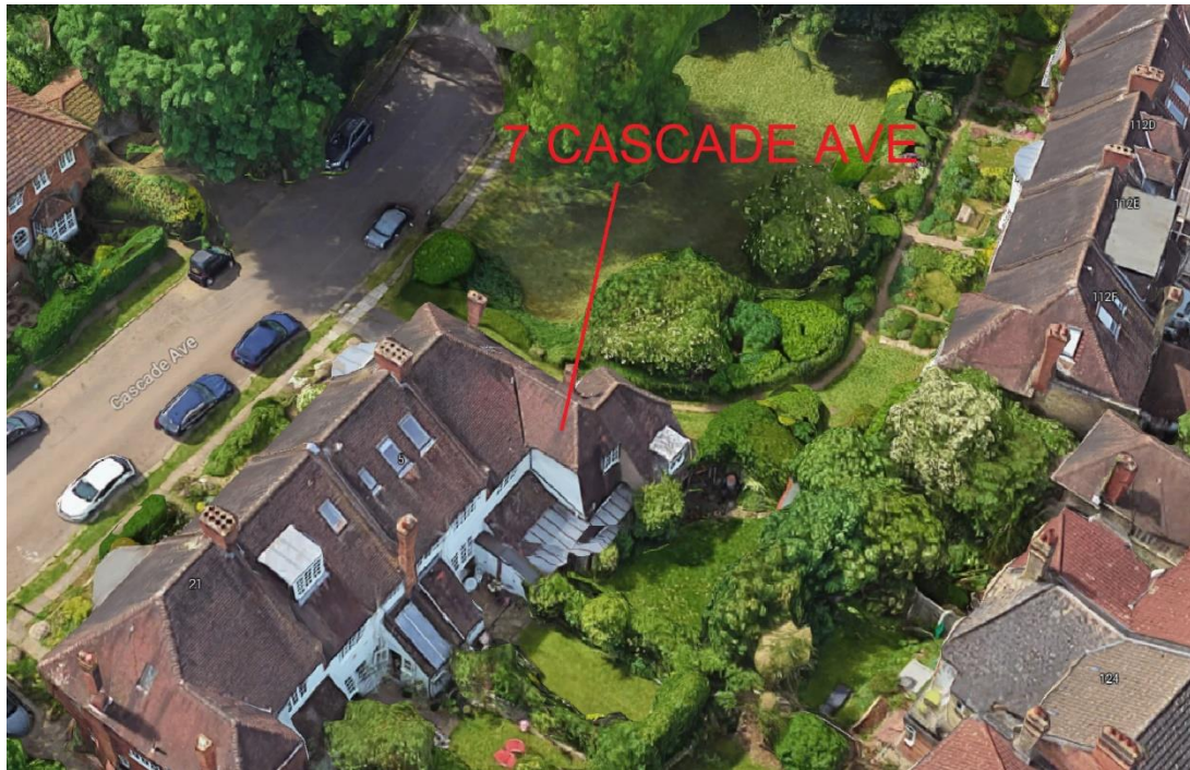
REAR ELEVATION SHOWING SIMILAR DORMER WINDOW AT NO 3 CASCADE AVENUE
