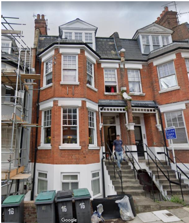
Front elevation of main property
