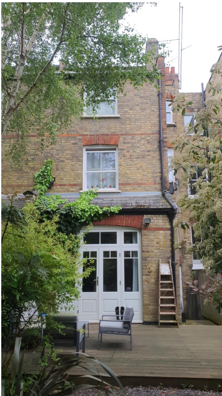
Rear elevation of main house
