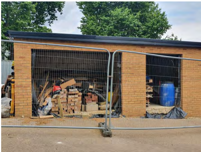
Abandoned bike/bin shed being used as a waste dump. Note blue chemical drum.
