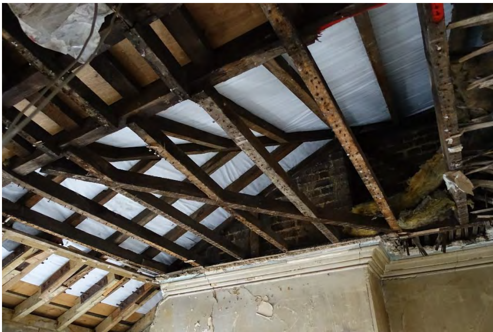
Views of ceiling and roof structure at 2 nd floor level: Note modern repairs to valley beam and to front gutter.
