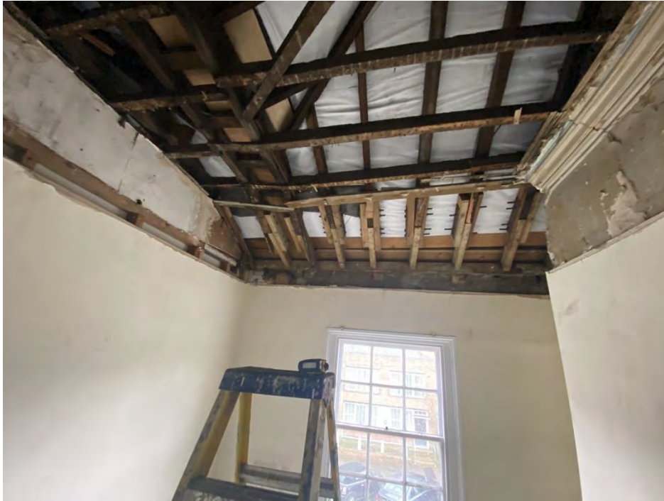
Views of ceiling and roof structure at 2 nd floor level: Note modern repairs to valley beam and to front gutter.
