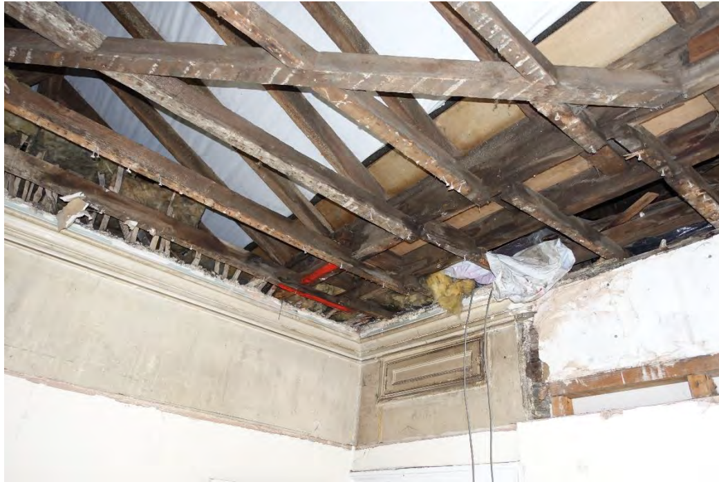
Views of ceiling and roof structure at 2nd floor level: front wall LHS
